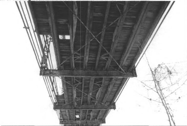
Photo 0010. Detail of stringers, floor beams and bottom lateral braces.
