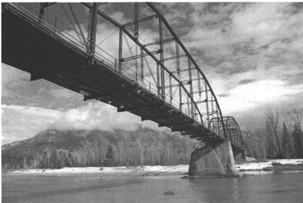
Photo 0004. West elevation of the Flathead River Bridge. View to the southeast.
