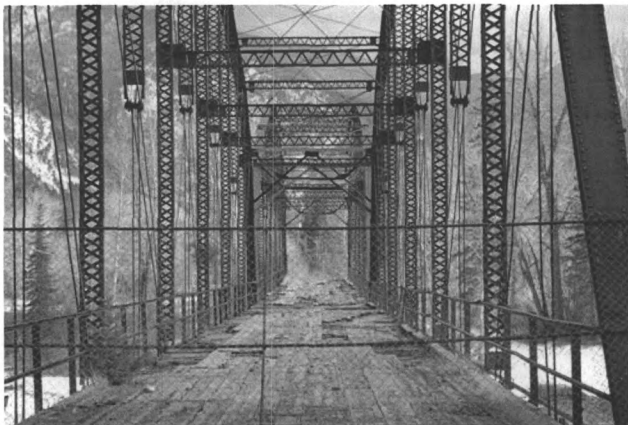
Photo 0009. Detail of existing deck and trusses. View to the west.
