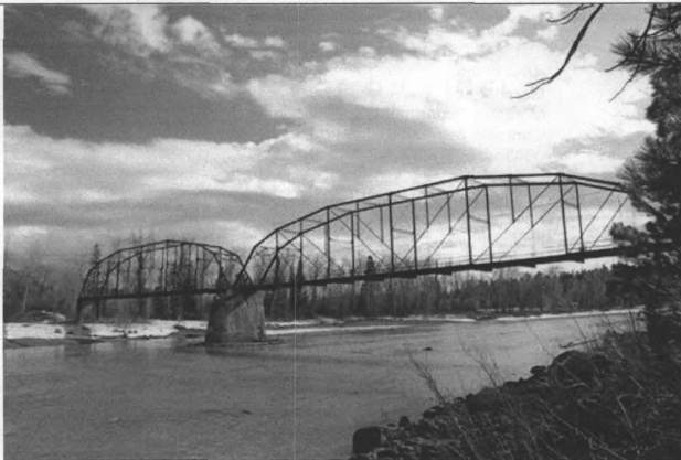
Photo 0001. East elevation of Flathead River Bridge. View to the southwest.
