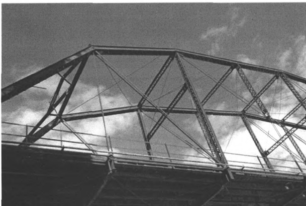
Photo 0008. Detail of steel superstructure of Flathead River Bridge.
