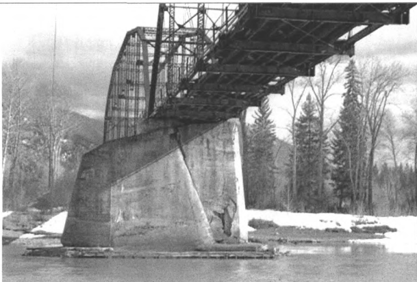
Photo 0007. Detail of concrete pier of bridge. View to the south-southwest.
