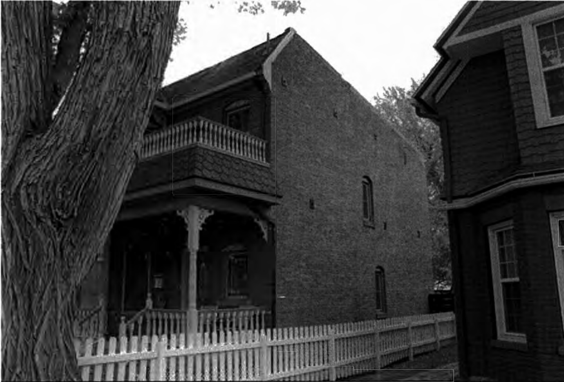
Photo 0004: North and west elevations, view to the southeast.
