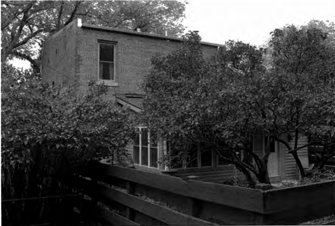
Photo 0008: South elevation, view to the northeast.
