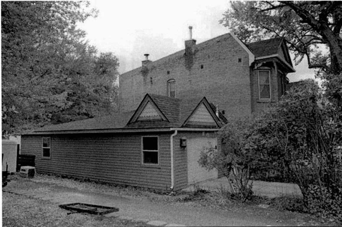
Photo 0005: West elevation, view to the southwest.
