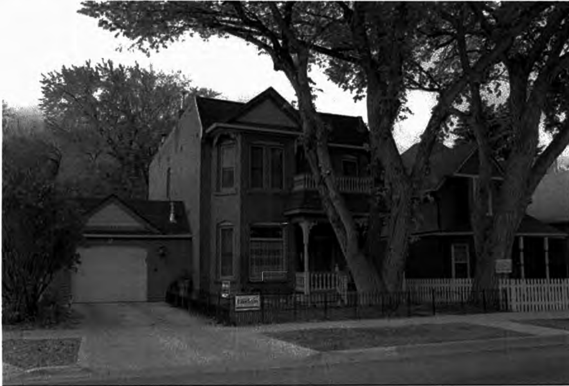
Photo 0002: North elevation, view to the south-southwest.
