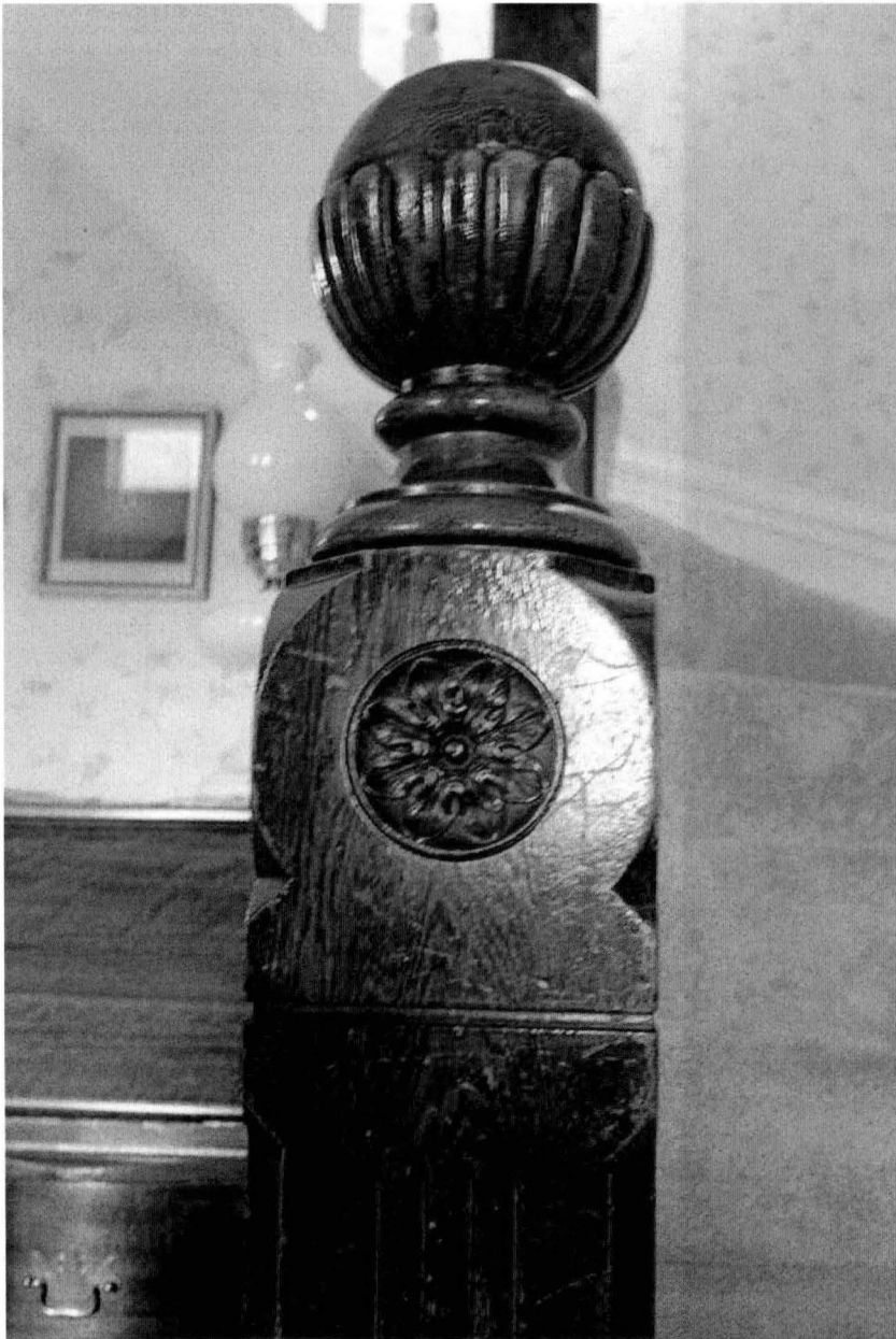
Interior detail of staircase.
