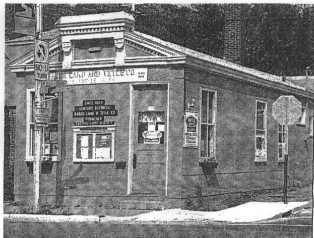
View of the Cushing Land Agency Building prior to restoration, 1998 (From "Preservation of a Landmark, Northern Currents The Leader , July 15, 1998.)
