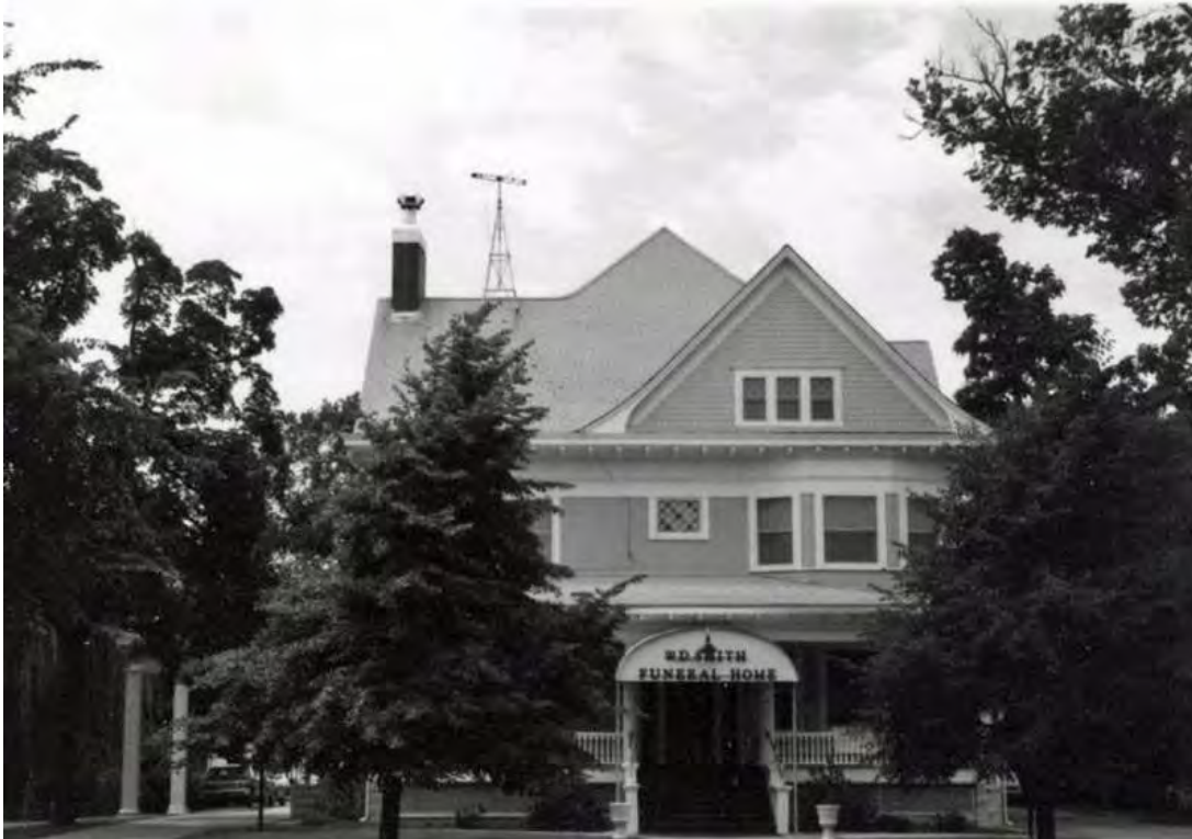
Figure 9. Circa 1977 photograph of east façade.
