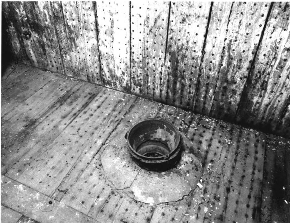
WEBSTER COUNTY JAILS PRESTON, WEBSTER CO., GEORGIA PHOTO 23 OF 23
