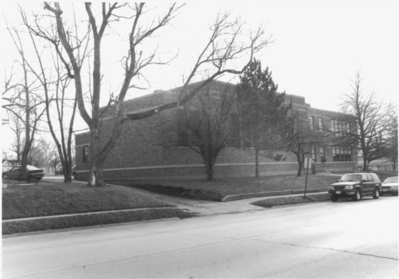
G. JEFFERSON ELEMENTARY SCHOOL: CRESTON, IOWA
