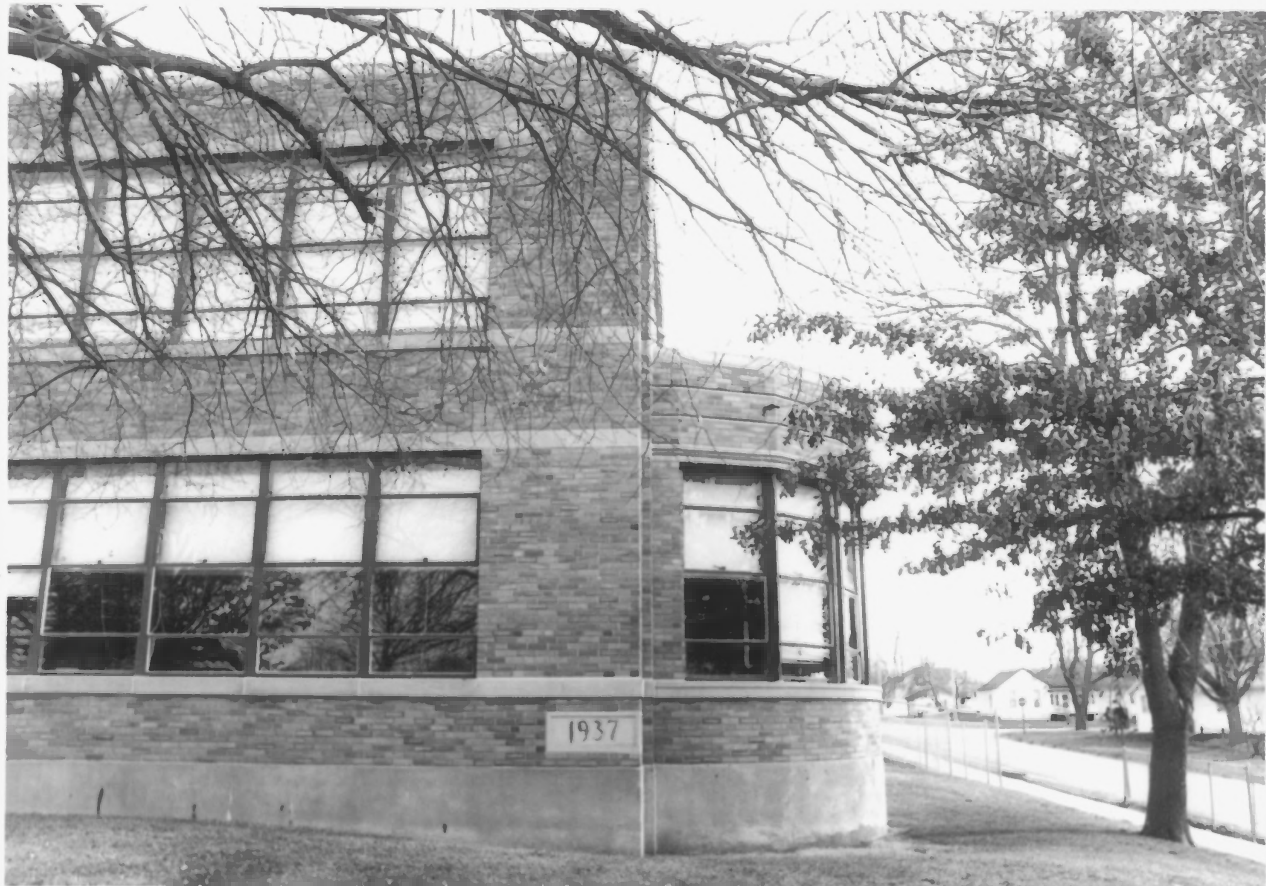
3. JEFFERSON ELEMENTARY SCHOOL: CRESTON, IA
