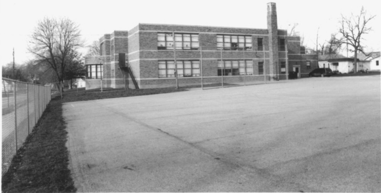
4. JEFFERSON ELEMENTARY SCHOOL, CRESTON, IOWA
