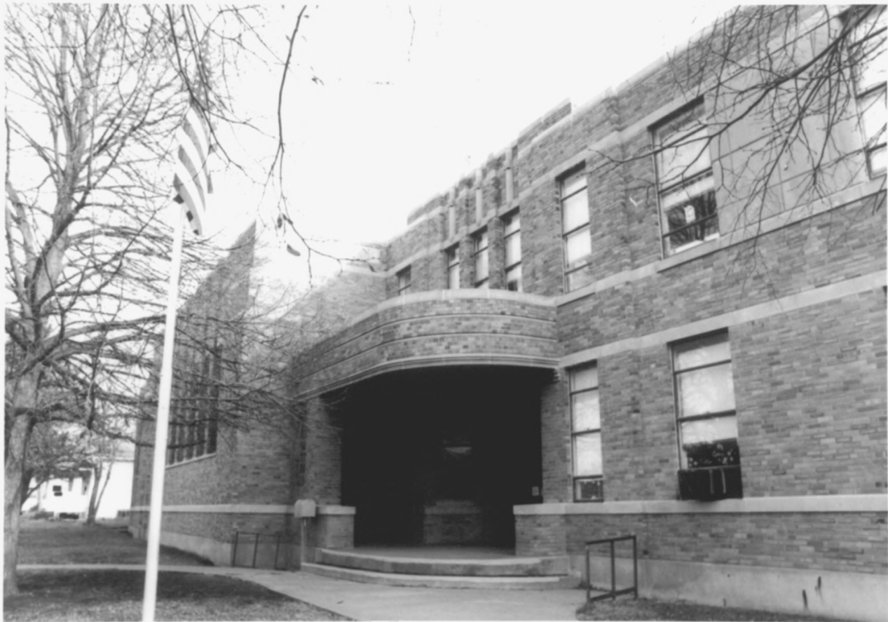
Z. JEFFERSON ELEMENTARY SCHOOL: CRESTON, IOWA
