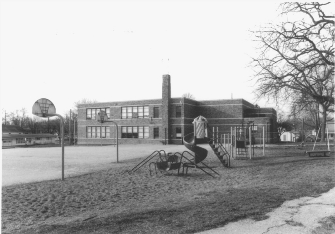
5. JEFFERSON ELEMENTARY SCHOOL: CRESTON, IOWA
