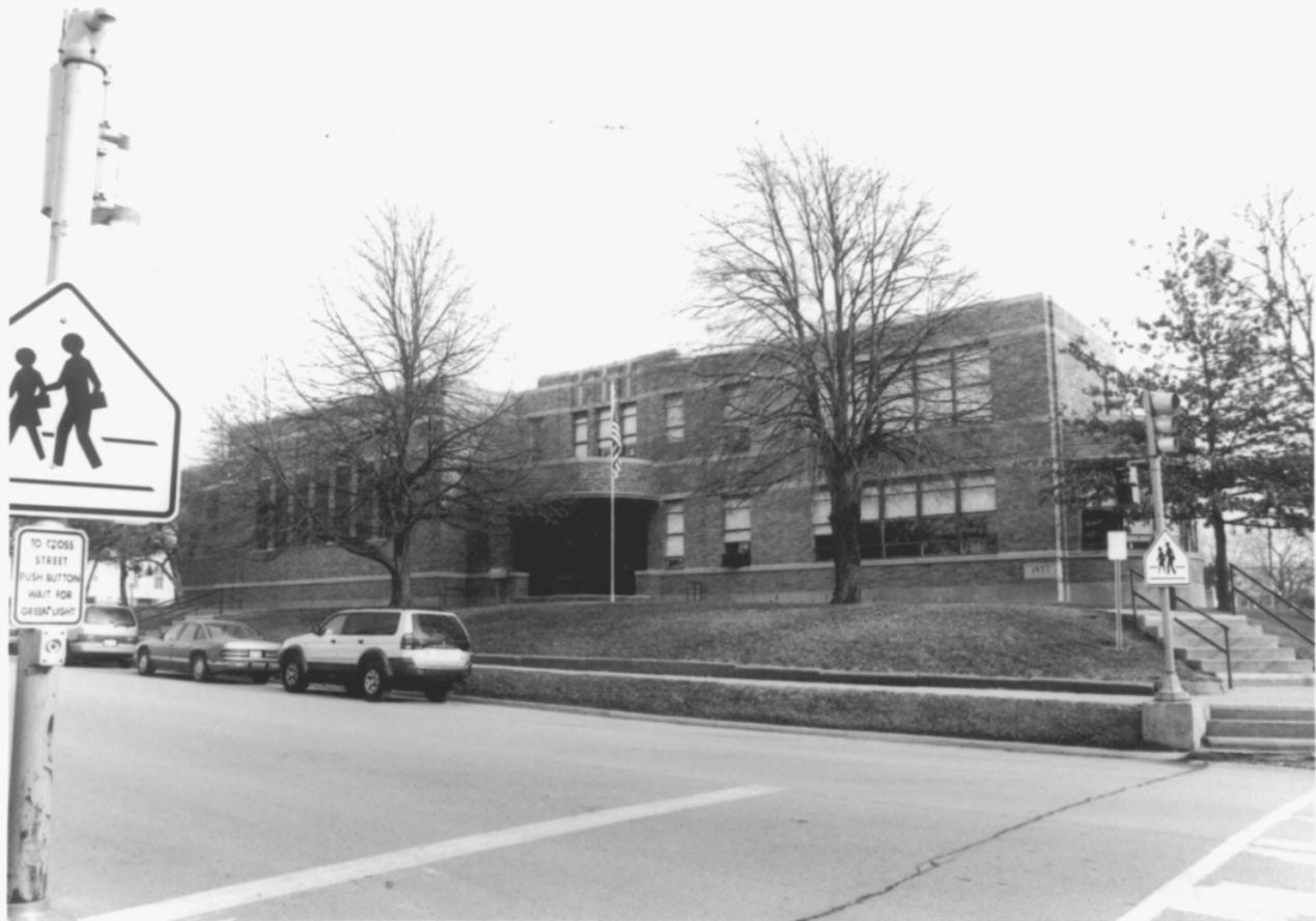
1. JEFFERSON ELEMENTARY SCHOOL: CRESTON, IOWA
