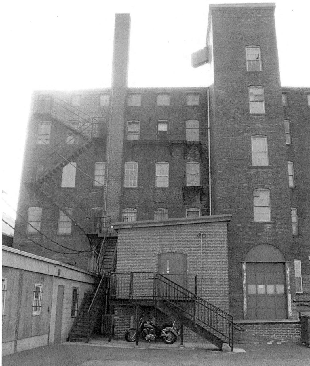
North (rear) elevation of factory from rear lot, showing elevator tower, chimney, fire escape, and rear ell details.
