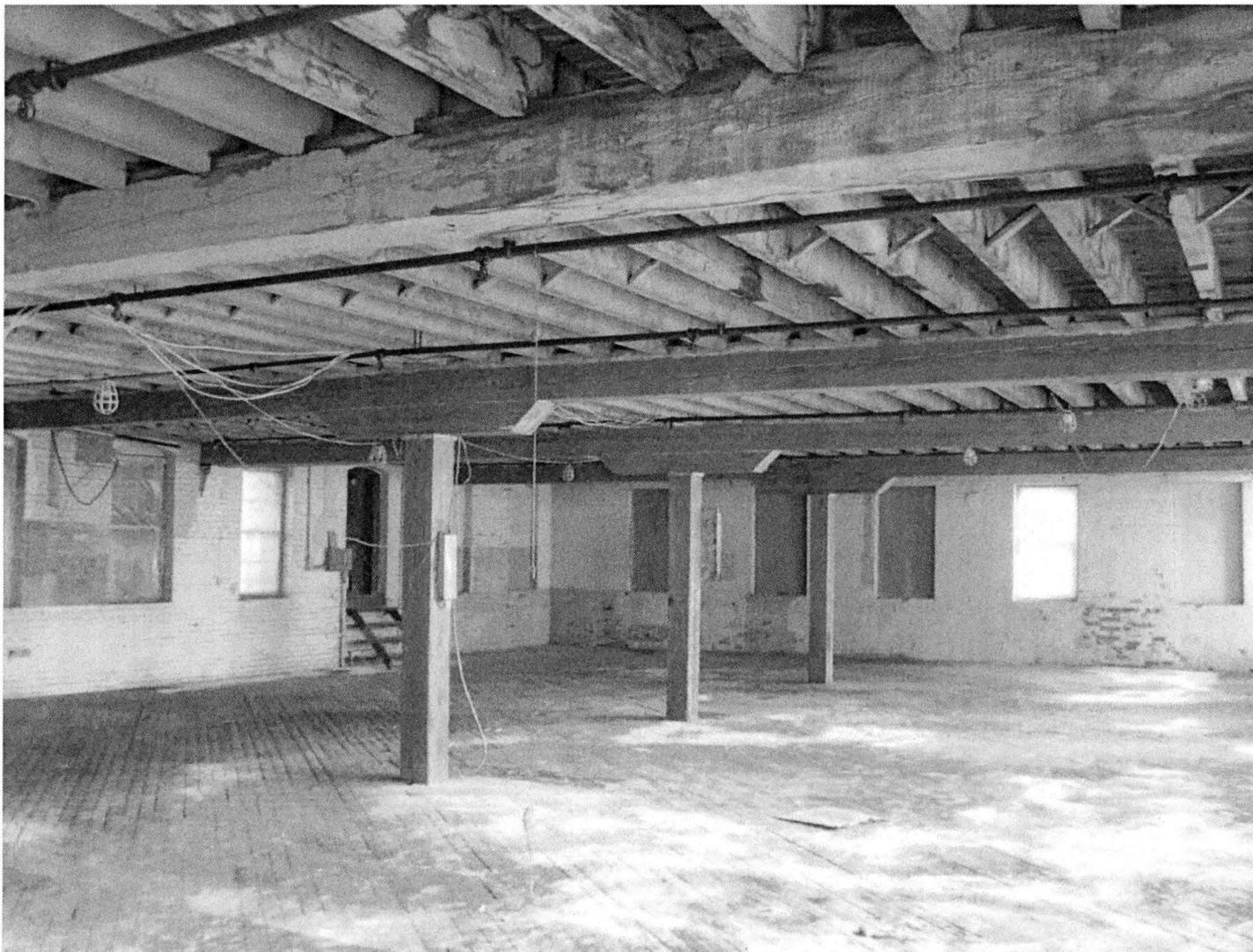
**Interior of the second level, showing typical upper-story details including fireproof floor, brick masonry walls, wooden posts, cross beams, and floor joists above.**
