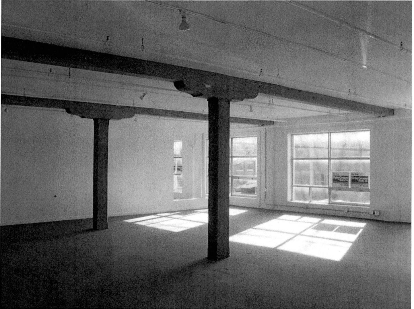
**Interior of the first floor showroom, showing details of the south (front) elevation fenestration, support posts, and cross beams.**
