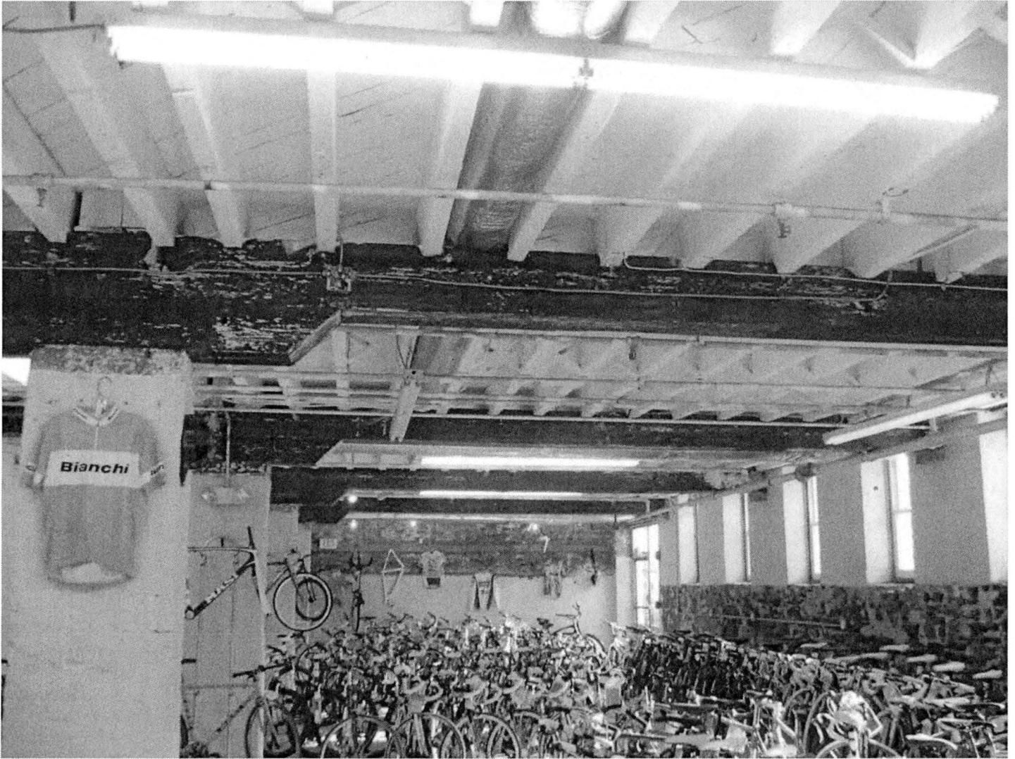
**Interior of basement level, showing details of the exposed foundation, brick support piers, cross beams, and floor joists.**
