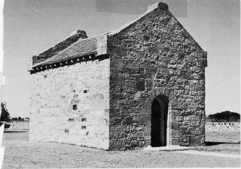
The powder magazine at Fort Belknap, an original structure, now houses a small chapel. National Park Service photograph.
