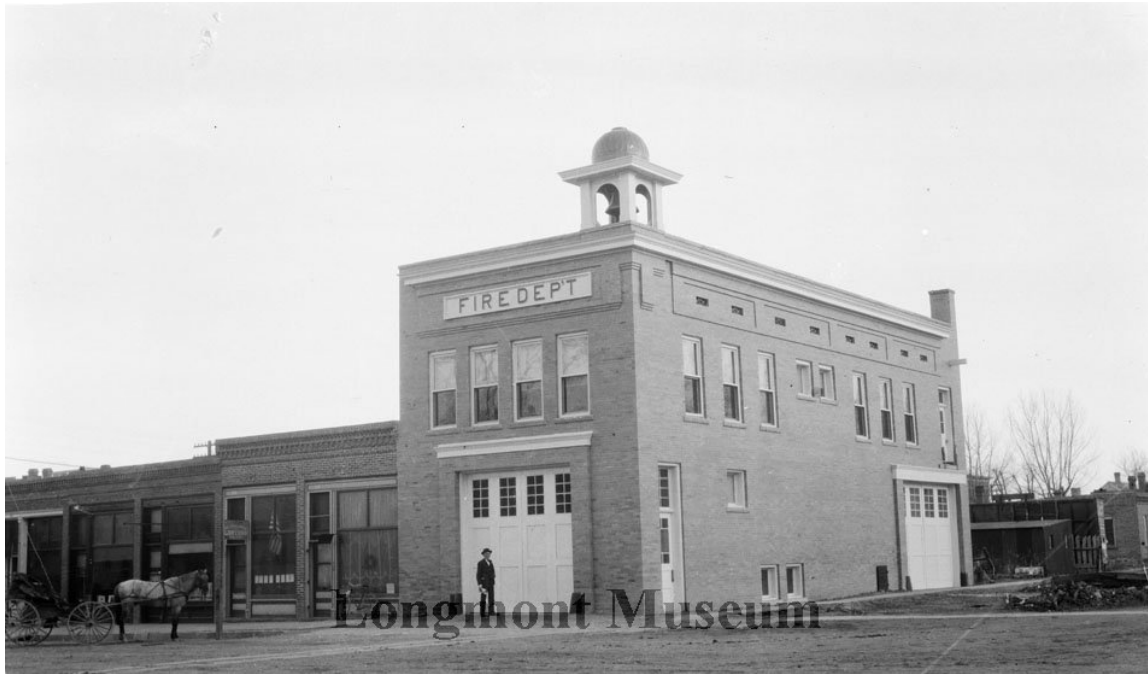
Figure 3: 659 4 th Avenue, 661/665 4 th Avenue, 667 4 th Avenue (Longmont Fire Department), view to SE, ca. 1907, courtesy Longmont Museum Archives, 2003.016.157.
