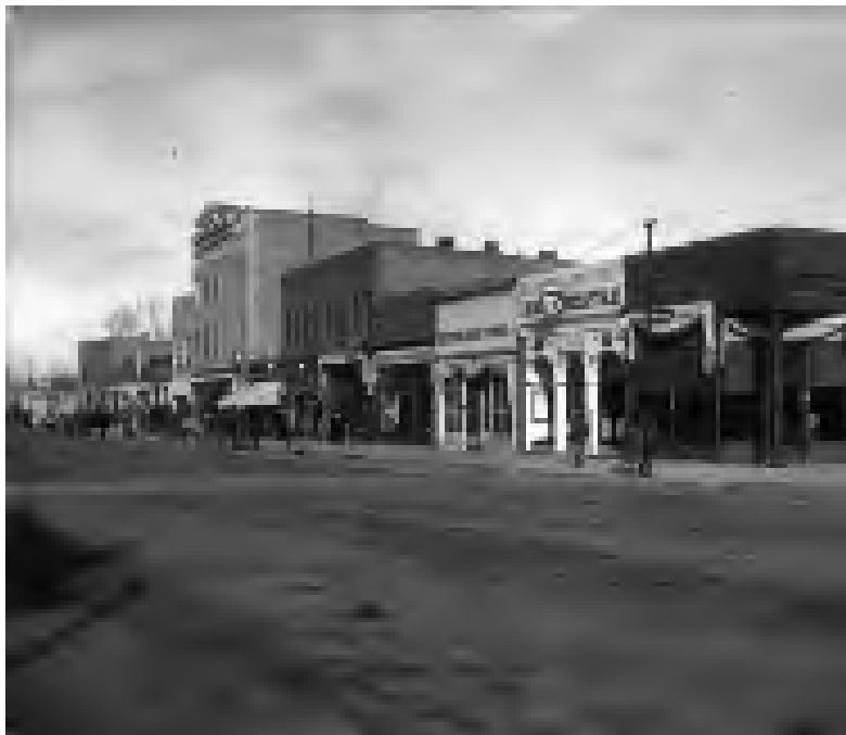
Figure 5: east side of 400 block of Main Street, view to NE, ca. 1910, courtesy Denver Public Library, x-10339.
