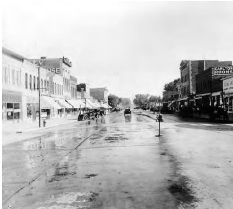
Figure 7: 400 block of Main Street, view to north, ca. 1920, courtesy Denver Public Library, x-12176.
