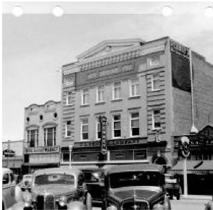
Figure 10: 430/434 Main Street (I.O.O.F. Building), 1941, view to NE, courtesy Longmont Museum Archives, 196.015.001.
