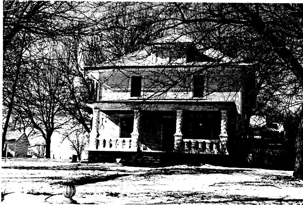
Building 20, View to the West.
