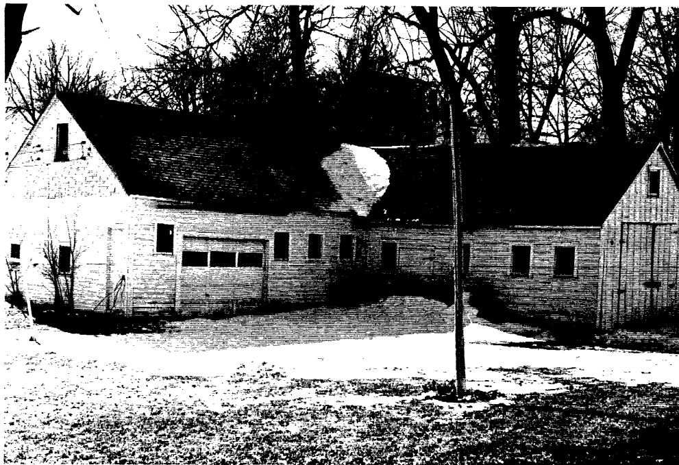
Horse Barn/Blacksmith Shop of Building 17, View to the WSW.
