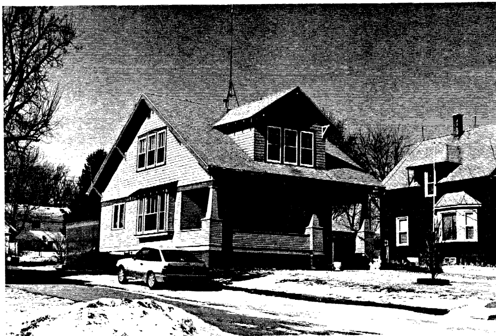
Building 36, View to the NW.
