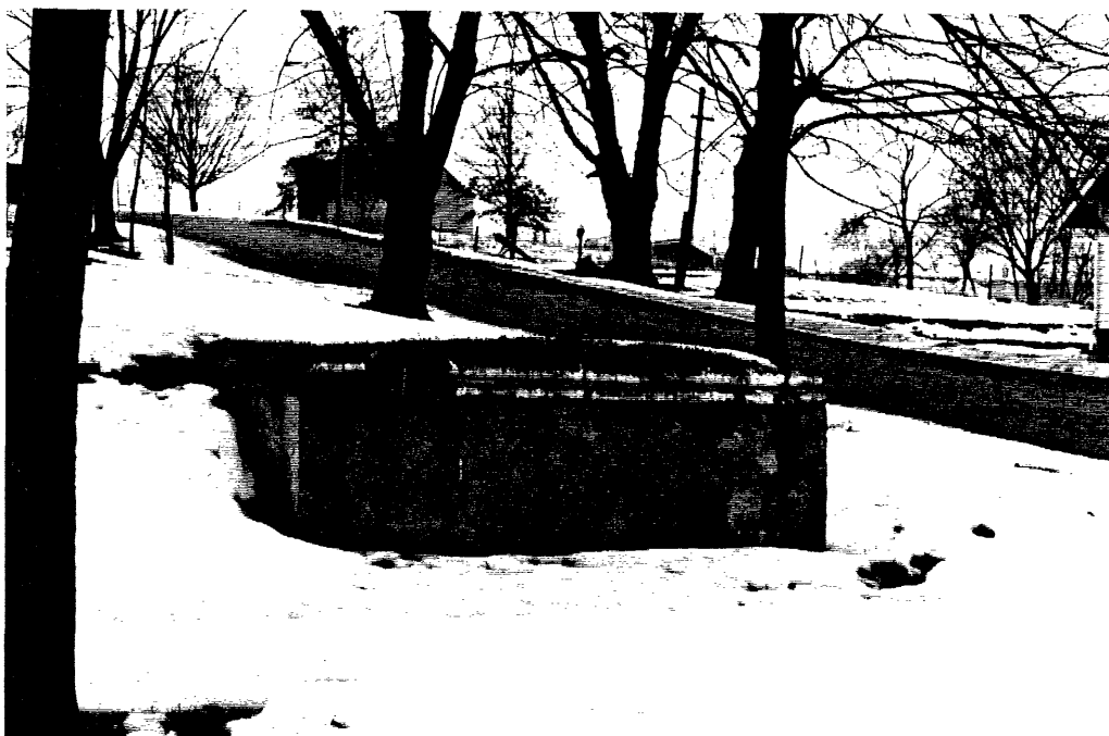
Photo 7-13. Object Types, Retaining Walls/Stairs, Building 20.
