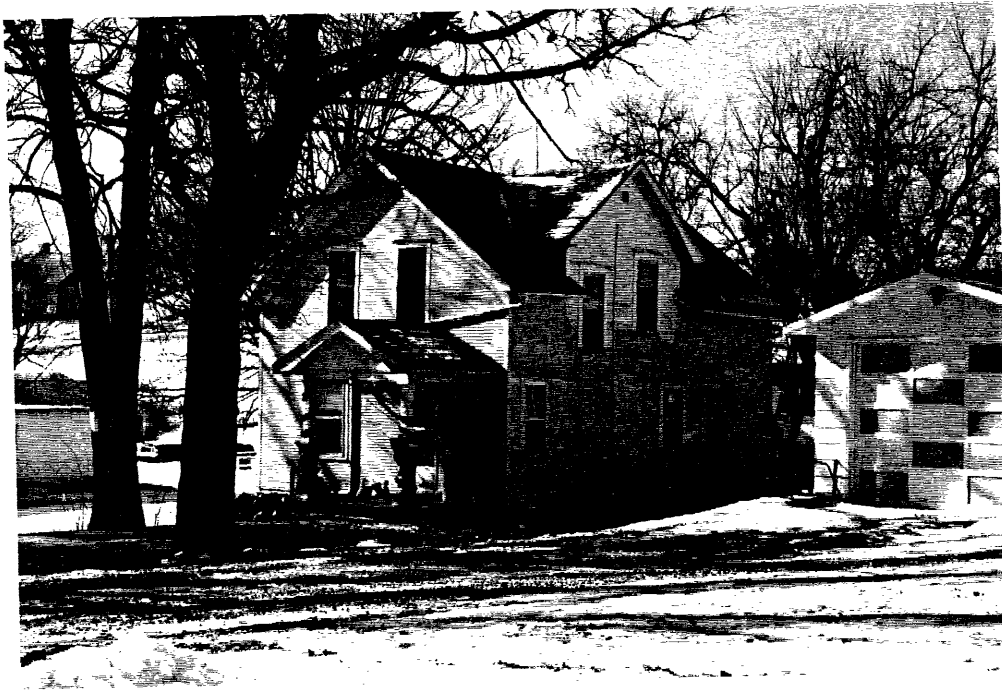
Building 17, View to the SW.
