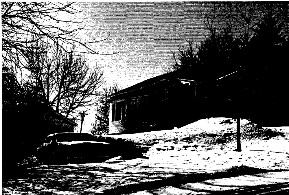
Building 21, View to the SW.
