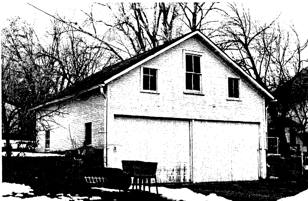
Garage of Building 25, View to the NNE.
