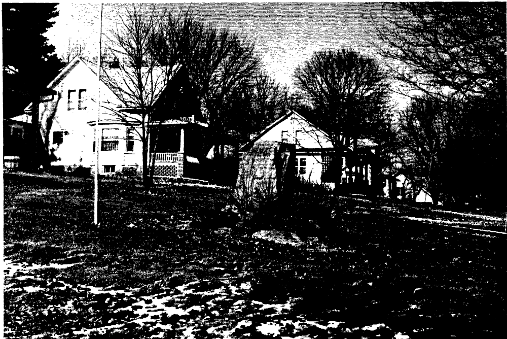
Boulder Marker, Building 24, View to the NW.
