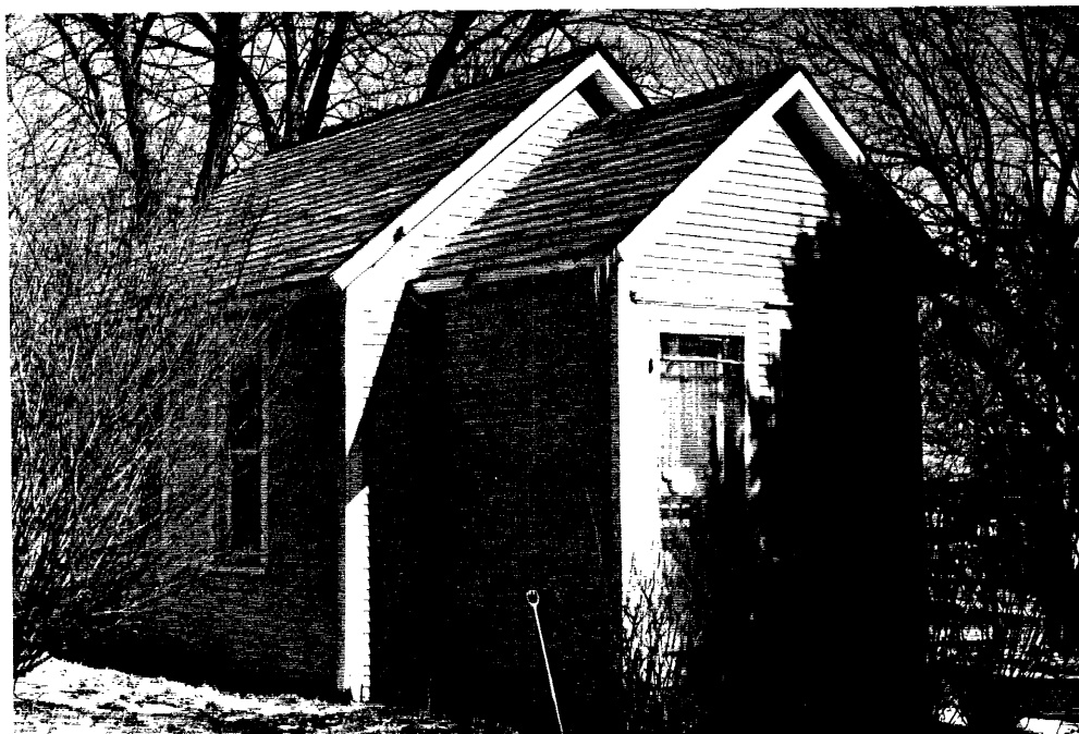
Grandfather's House of Building 22, View to the NE.
