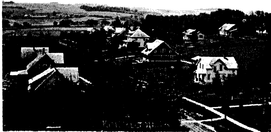
View of Buildings 3, 5, 17-25, taken c.1922, View to the SW.
