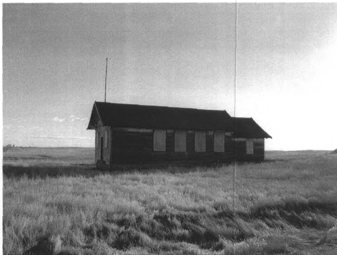
1. Overview of school, view to southeast
