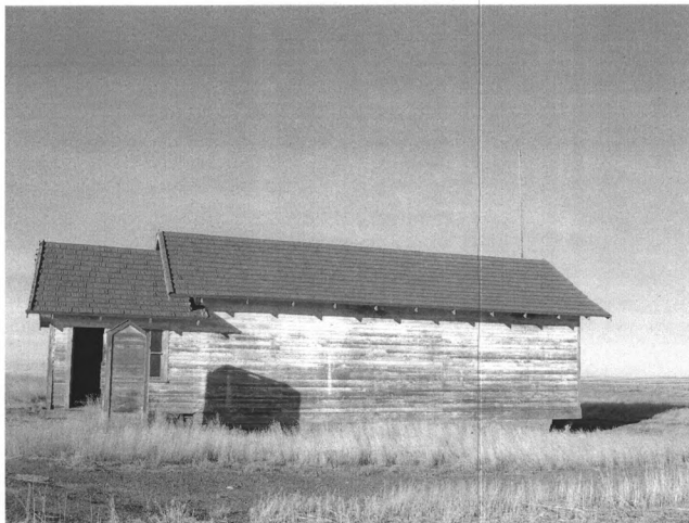
5. School, east elevation, view to west
