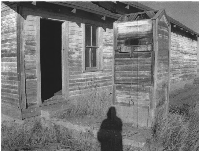
6. Cistern, south and east elevation, view to northwest
