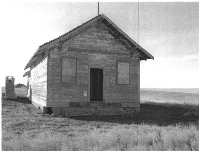
2. School, façade (north elevation), view to south
