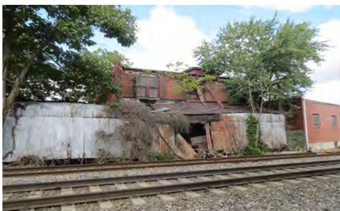
View of Southeast facade
