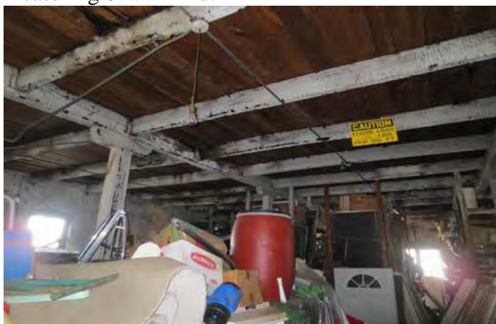
Interior, Second Floor
