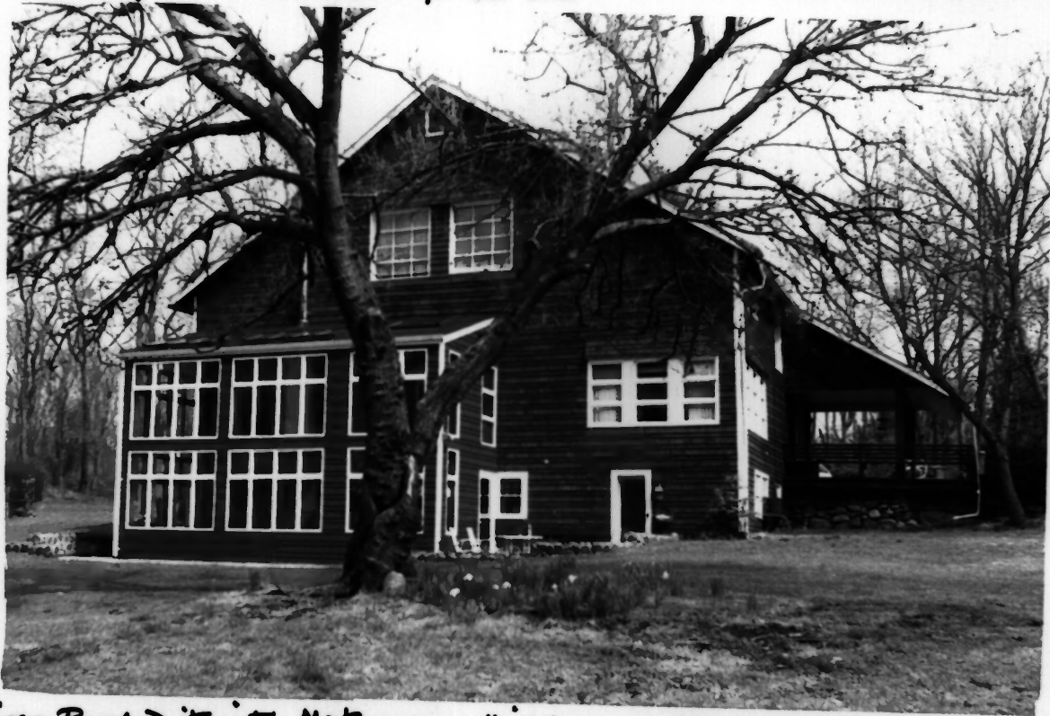
River Road District, Montgomery-Hillsborough Towns, Somerset Co., N.S.
