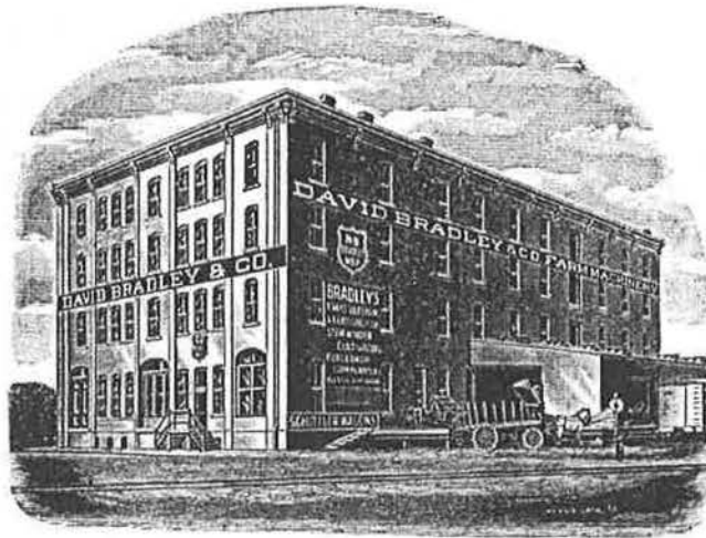
Figure 13: Bradley David and Company at 1100-1116 South Main (non-extant), 1906.
