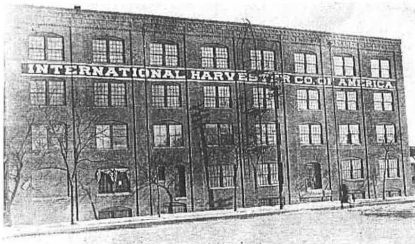
Figure 16: McCormick Harvesting Machine Company Building at 1001 South 6 th Street, Date Unknown. (NRN Ref. 12000780, Listed 9/10/2012)
