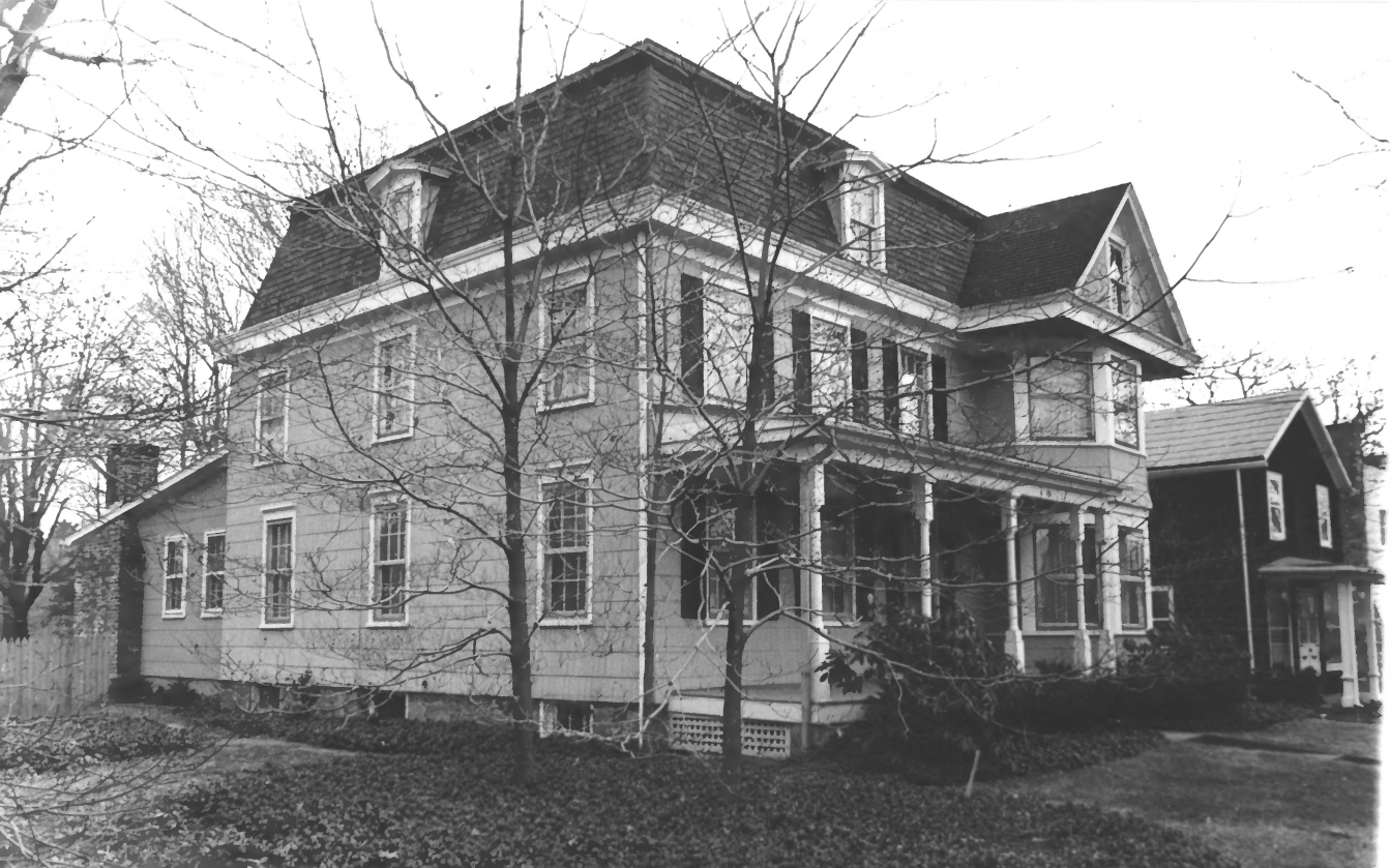
13 + 11 MOUNTAIN AVE. MENDHAM, N.J. PHOTO 1983 JWF/ROLL 5 NEG. 15
