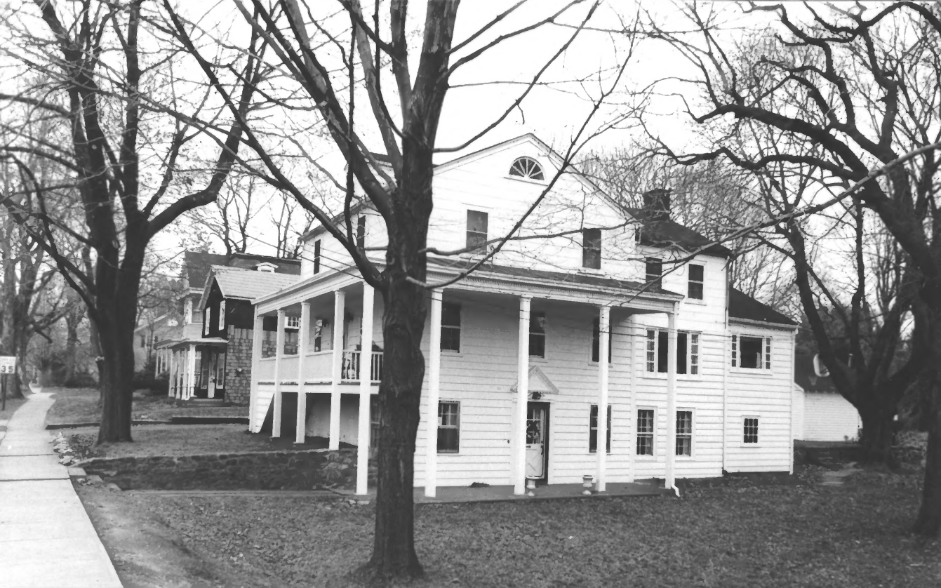
9 MOUNTAIN AVE. MENDHAM, N.J. PHOTO 1983 JWF/ROLL 5 NEG. 22
