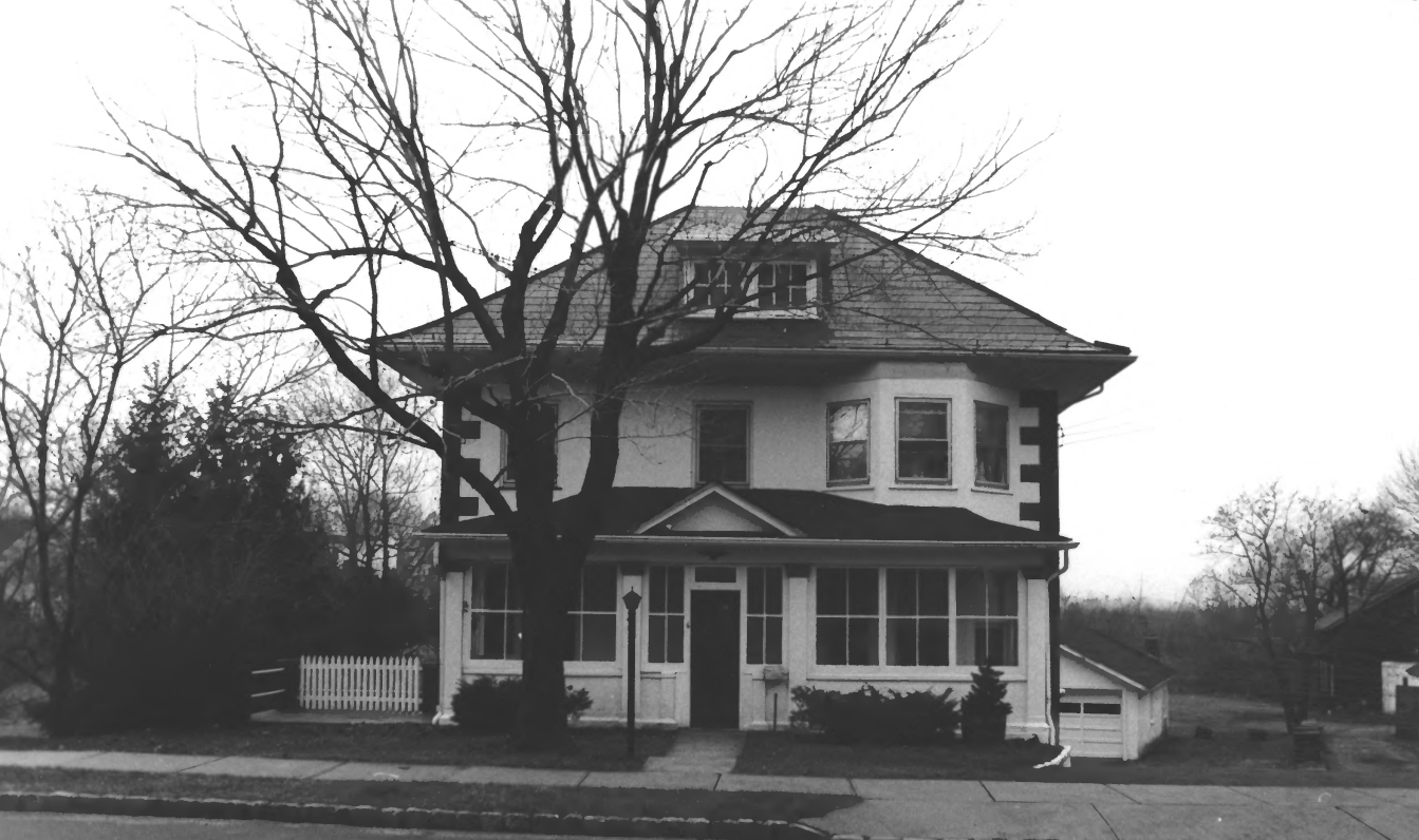
6 MOUNTAIN AVE, MENDHAM, N.J. PHOTO 1983 JWF / ROLL 5 NEG. 23
