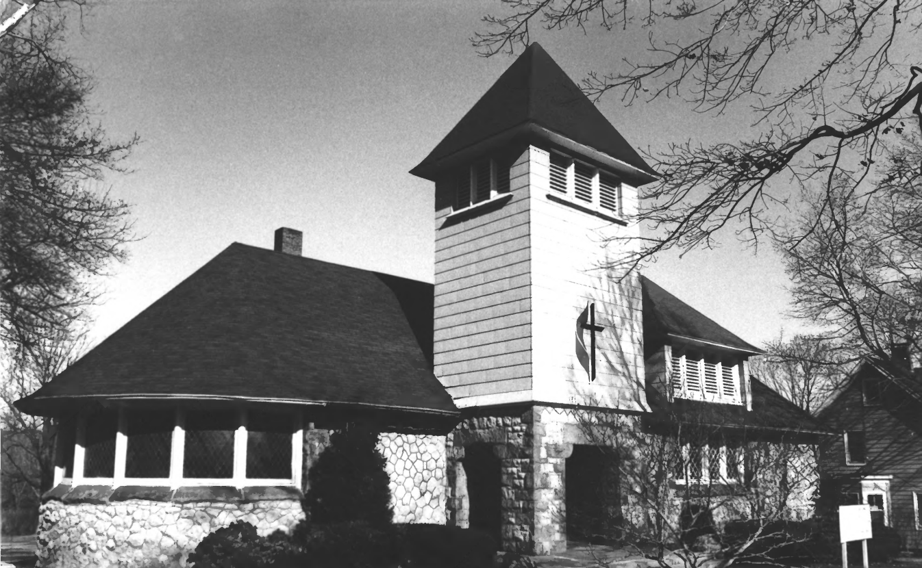
MENDHAM METHODIST CHURCH 10 EAST MAIN ST., MENDHAM, N.J. PHOTO. 1983 JWF/ROLL 4 NEG. 19
