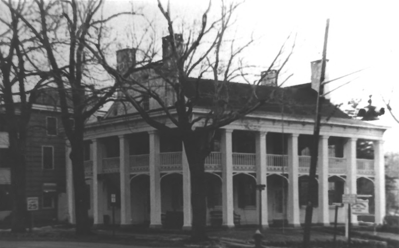
PHOENIX HOUSE 2 WEST MAIN STREET, MENDHAM, N.J. PHOTO ca. 1965 ROLL 8 NEG. 6 JWF 1-84
