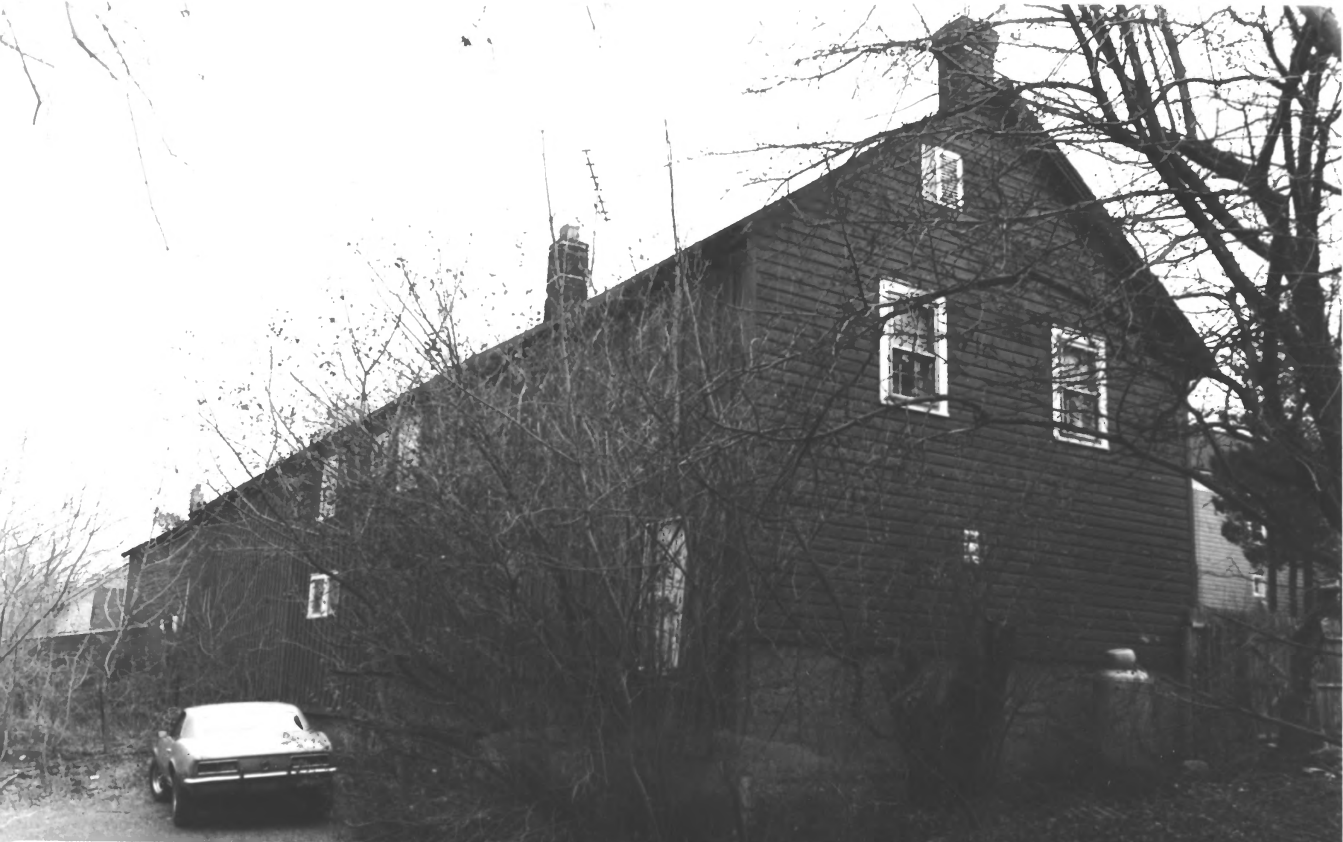
STABLES BEHIND #4 EAST MAIN ST. MENDHAM, N.J.
