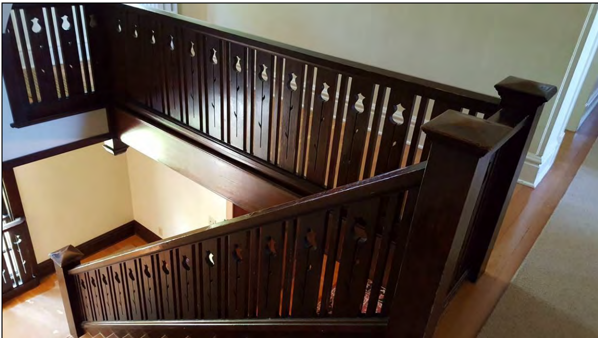
15 of 30 WA_Spokane County_Bleecker House_0015.tiff Staircase to second floor from reception hall in 2019
