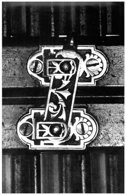
Joseph Shafer House Brookville, IN 47012 R.L. Wadsworth Jr. 8/80 Negative at house Brass interior shutter fitting (24 sets)
