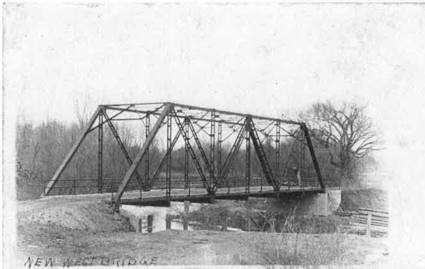
Figure 1: Undated early photo of West Bridge. Photo courtesy of the Watonwan County Historical Society.
