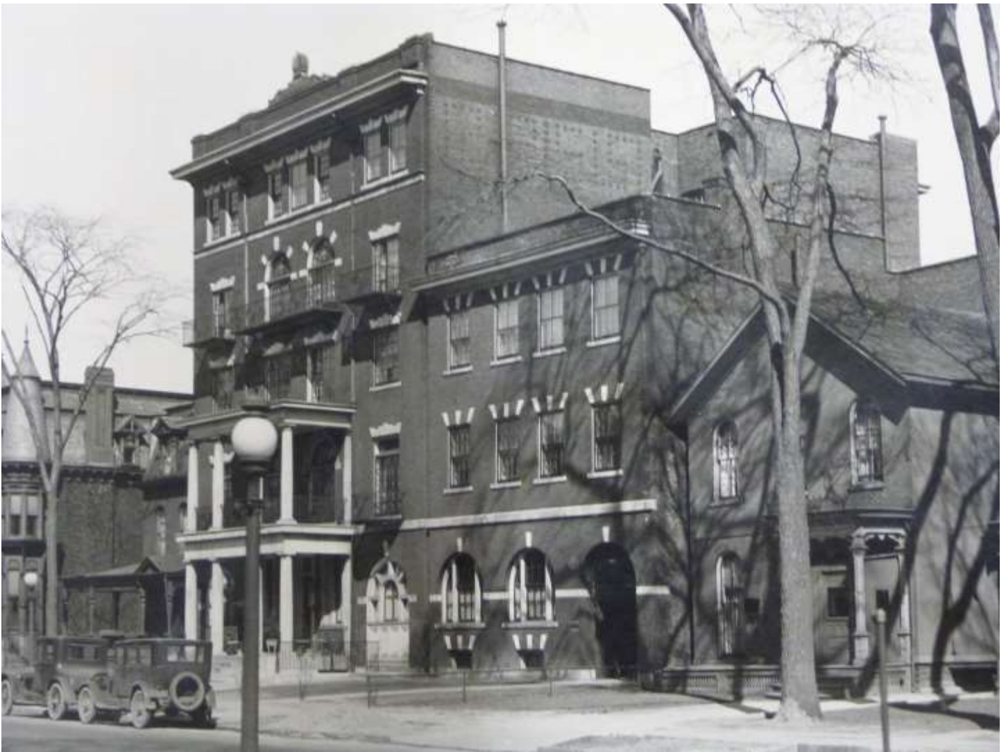
Historic Photograph 2. 1925 looking northeast showing The Colonial Flats (1896) by Boughton and Johnson to the north and The Colonial Annex (1900) by Esenwein and Johnson to the south. Note that the profile of the cornice on the east elevation (no longer extant) is visible. Photo is from a postcard located at the Buffalo History Museum. Reed Service Inc. Investment Realty. 4/25/1925 is noted on the back of the postcard.
