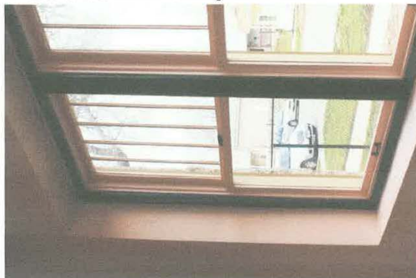
16 Interior East Windows Looking East 12/17/2012
