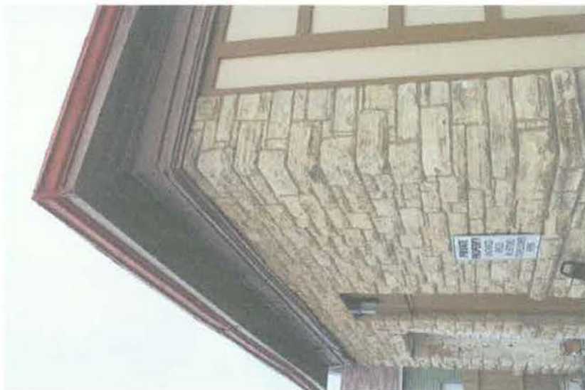
2 Cornice Detail Looking North East 12/17/2012
