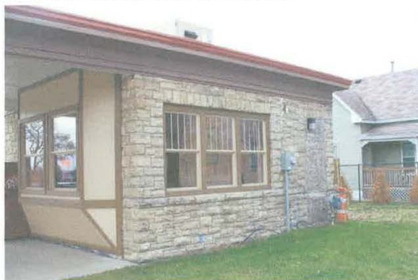
8 East Wall Looking North West 12/17/2012
