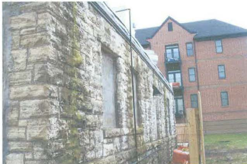
6 Back Wall Looking West 12/17/2012
