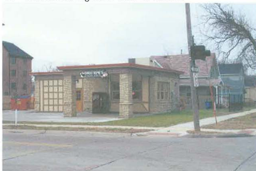
11 Exterior Looking North West 12/17/2012
