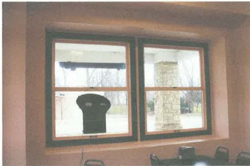
15 Interior South Window Bay Looking South East 12/17/2012
