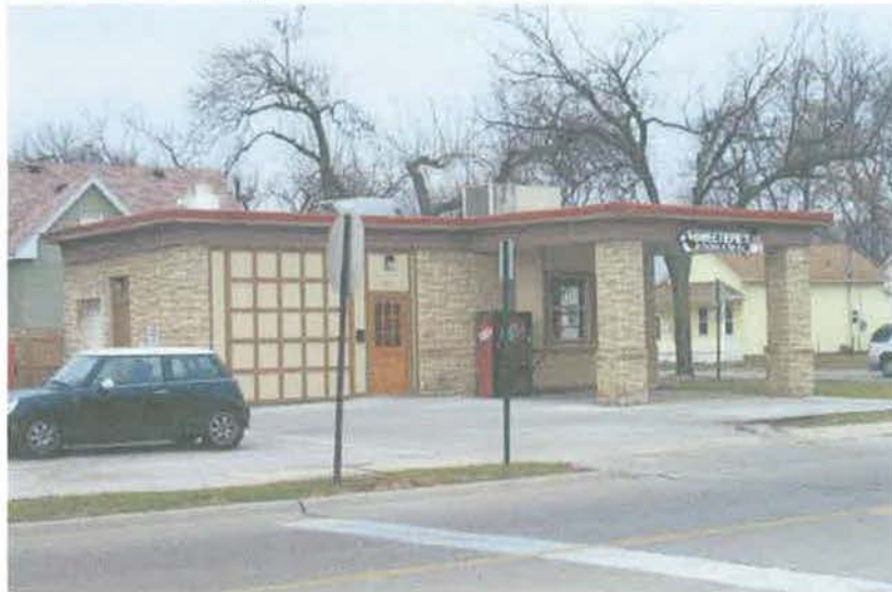
1 Facade Looking North East 12/17/2012
