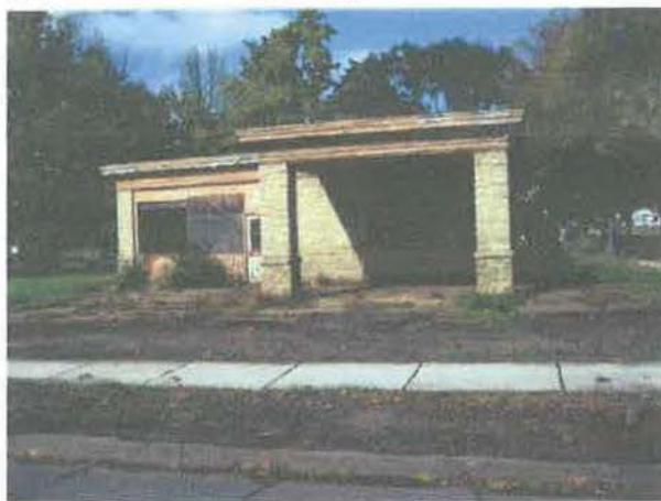
Figure 8b. View From South (Pre-Rehabilitation, 2011)
