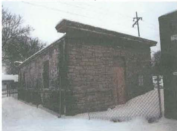
Figure 8c. View From West (Pre-Rehabilitation, 2011)
