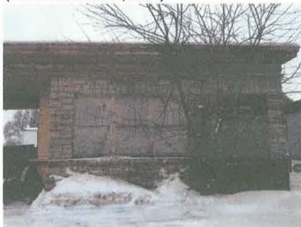
Figure 8d. View From North East (Pre-Rehabilitation, 2011)
