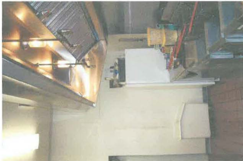
17 Interior Kitchen Looking North West 12/17/2012
