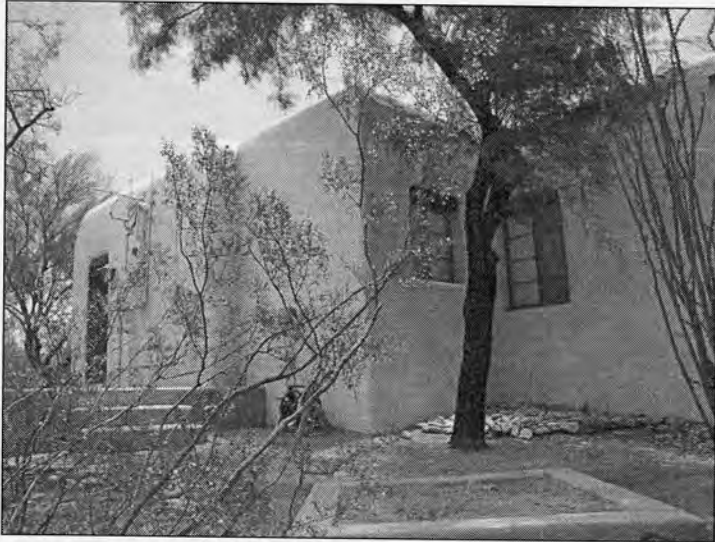
Photograph #5 West façade, camera facing northeast.
