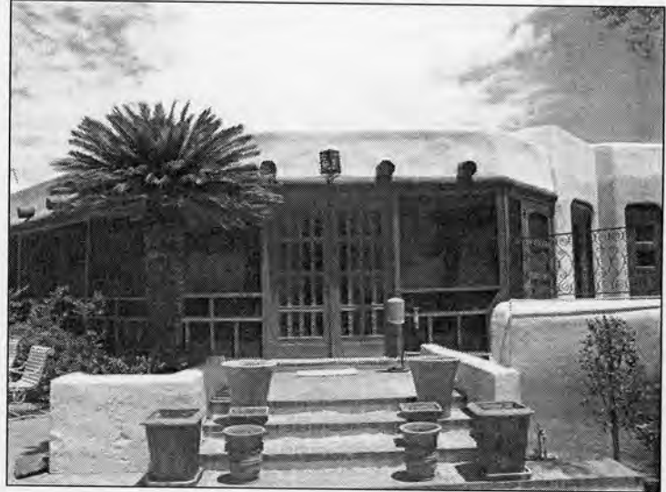
Photograph #2 Partial south façade showing screened porch, camera facing north.
