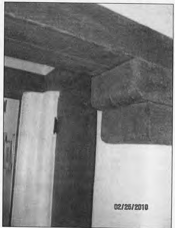
Photograph #8 Lintel detail, entrance to west wing hall, camera facing northwest.
