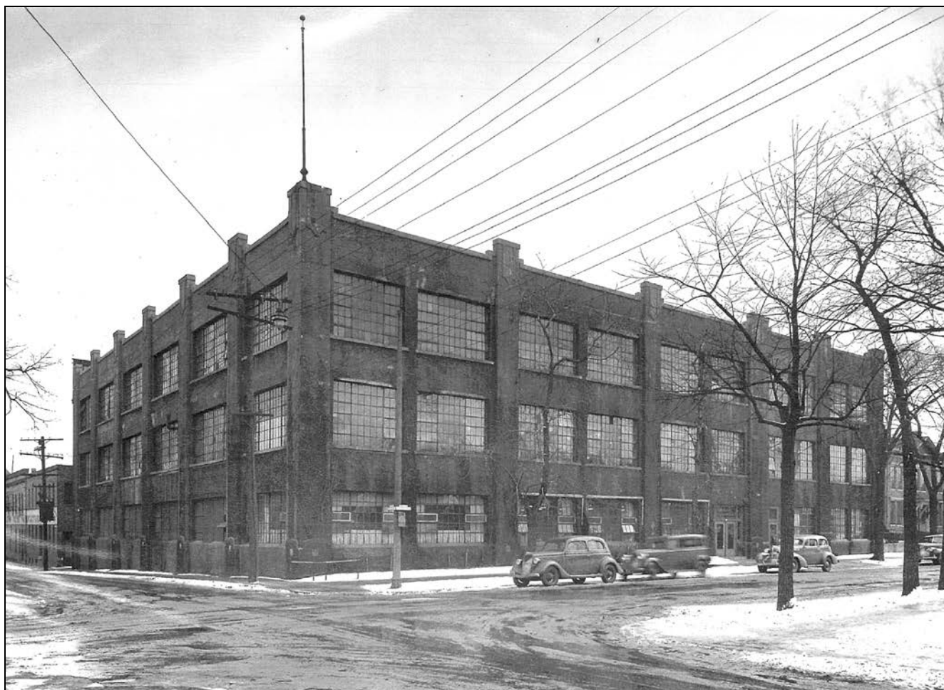
1940 historic photograph showing the primary (South 3 rd Street) and north (West Pierce Street) facades. [Photograph property of the Milwaukee County Historical Society (South 3 rd Street File), Milwaukee, Wisconsin]
