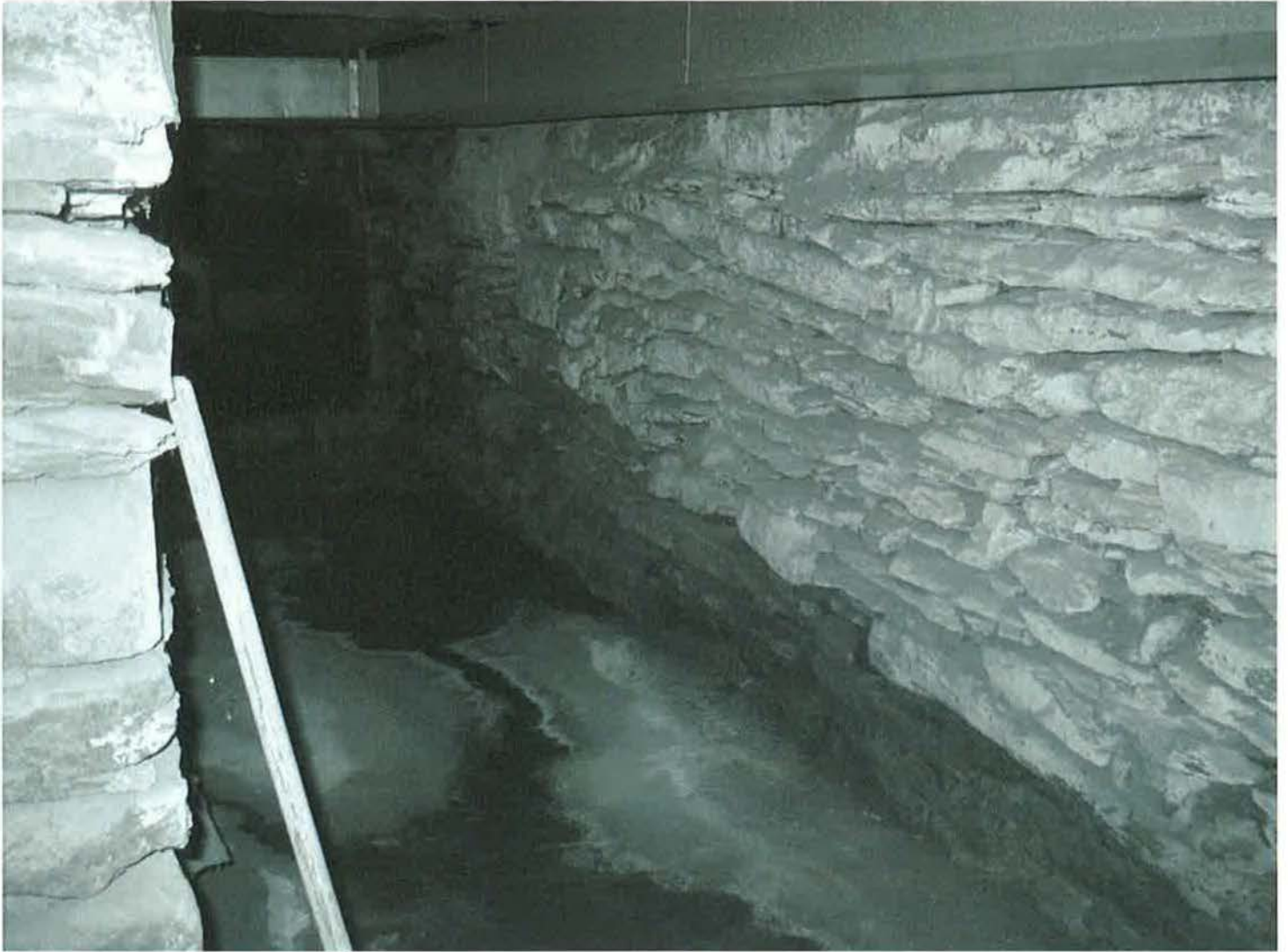
Interior of cellar, showing foundation detail. Camera facing northeast. Photograph 2 of 20.
