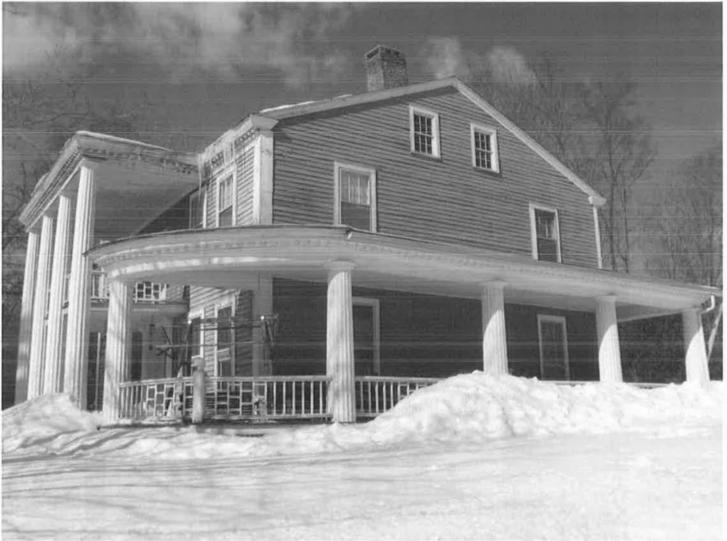
South (front) and east (side) elevations of house from Spoonville Road, showing side porch details.
