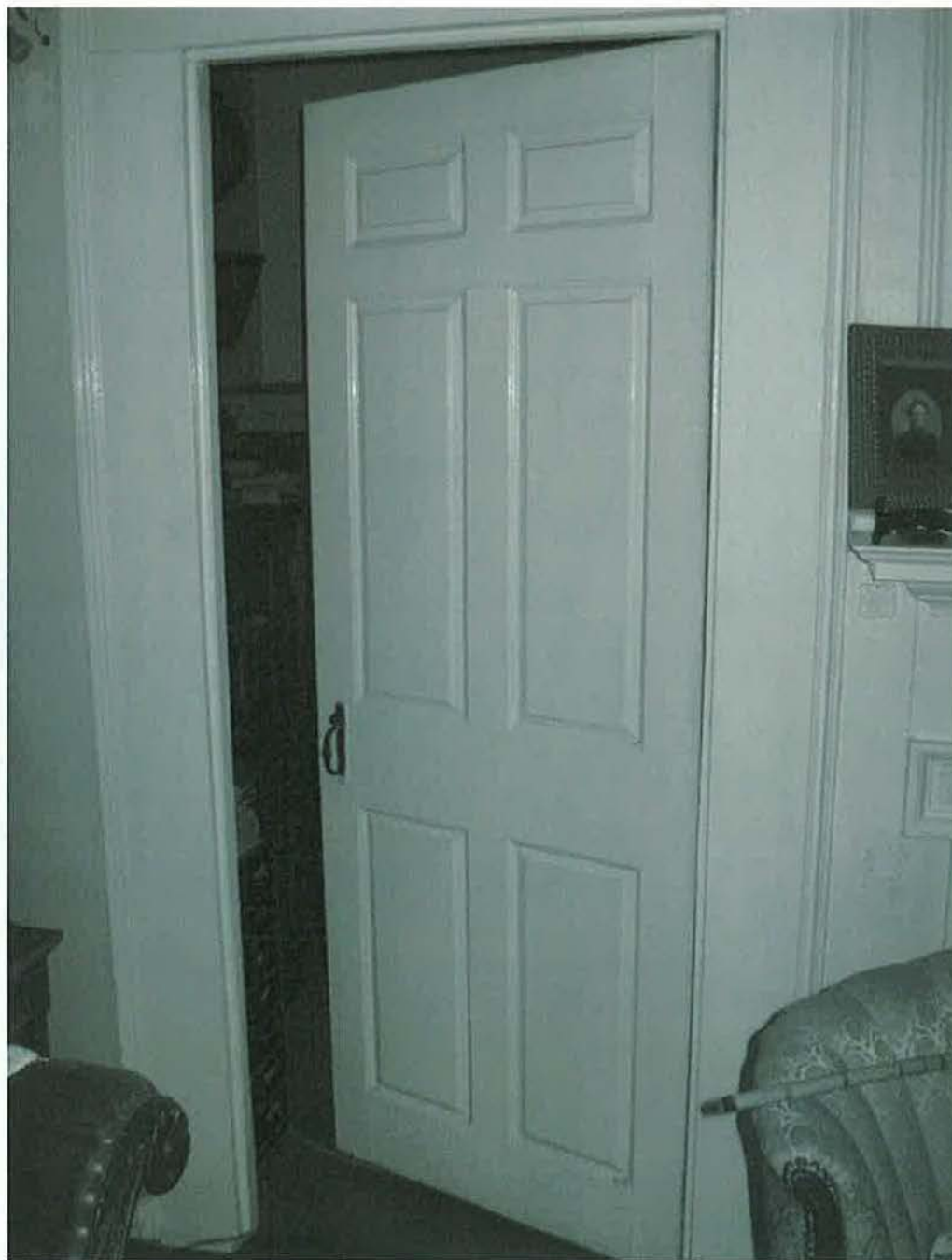
Interior of northeast chamber, showing six-panel door details. Camera facing southeast. Photograph 16 of 20.
