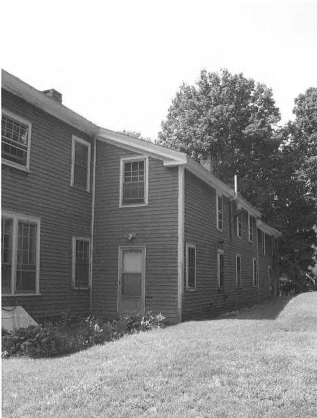
North (rear) and east (side) elevations of house from the "Old County Highway", rear lean-to details.
