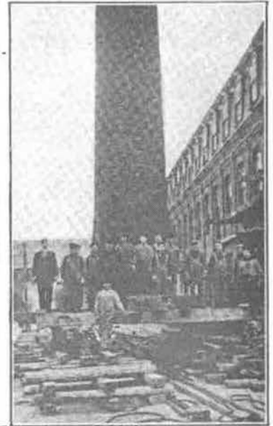
Figure 27. View of C. H. Brown buildings being moved in 1910, from "Moving a Brick Machine Shop," American Machinist , June 9, 1910.
