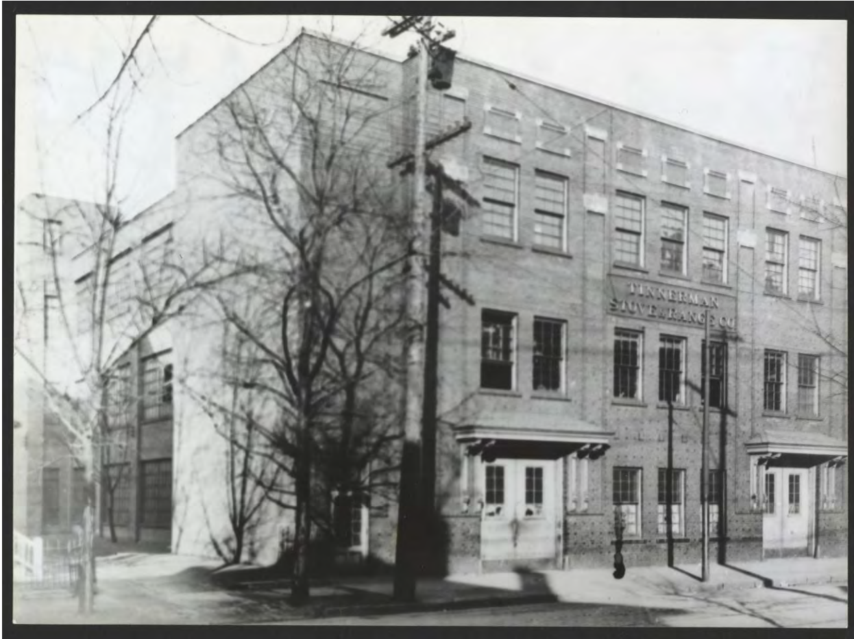
Figure 19: Historic photo of the south and east (front) elevations of the 1914 addition on Fulton, looking northwest, date unknown. Source: Cleveland Public Library Digital Collection, CP02759, Cleveland, Ohio.
