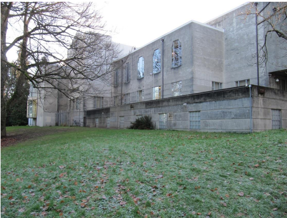
009 Oblique view looking southeast at the east façade.
