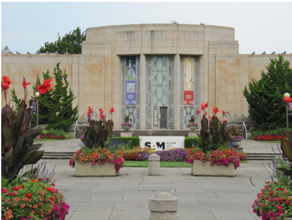
003 View looking east at the main entry on the primary (east) façade, stone paving and steps
