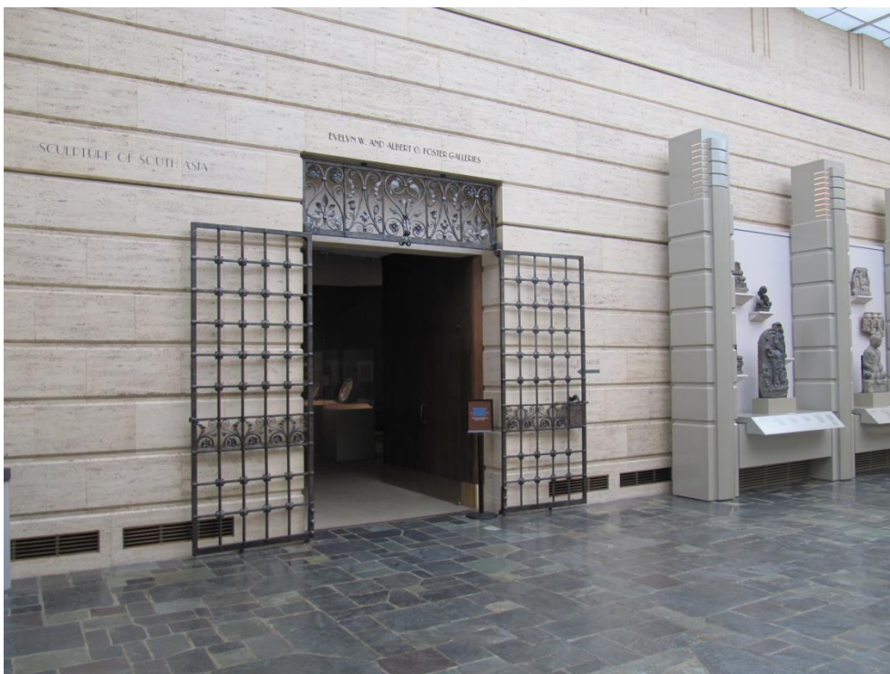
019 Detail view of ornamental bronze entry gate to galleries in the Garden Court
