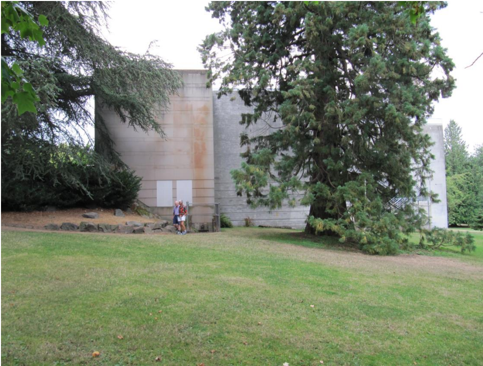
006 View looking north at the south facade
