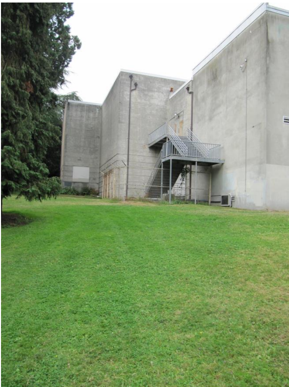
007 Oblique view looking northwest at the southeast corner
