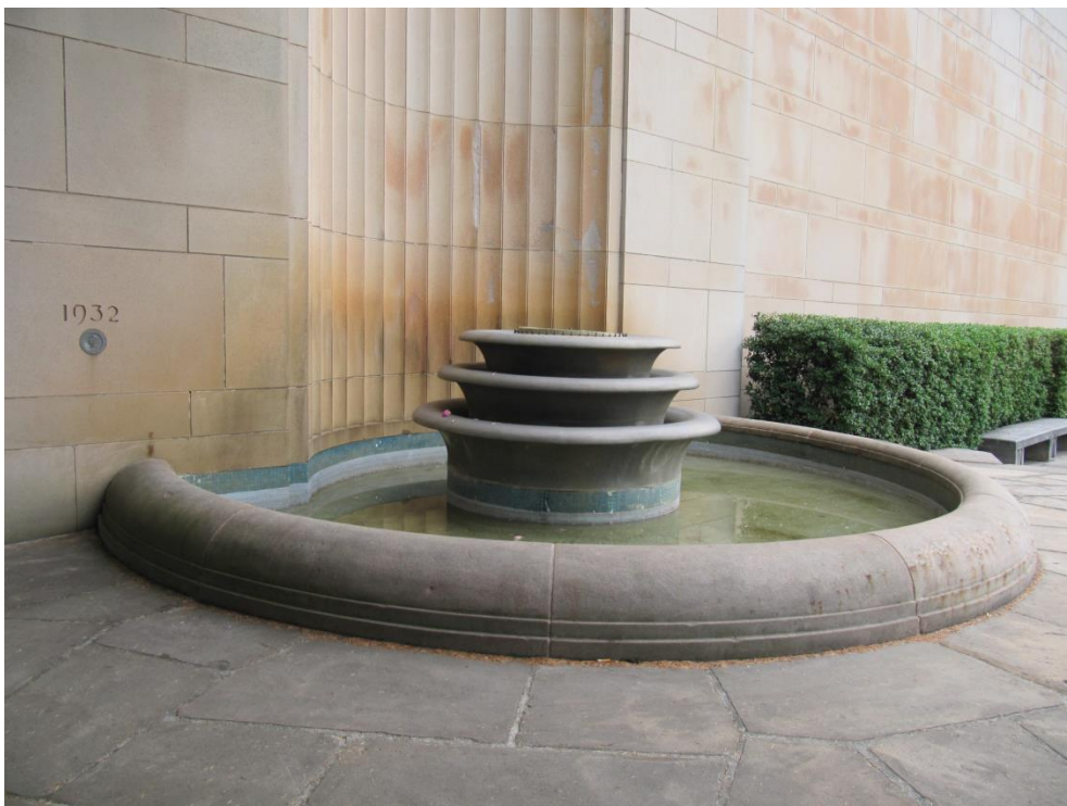
005 Detail view looking southeast at the pool near the north end of the primary (east) facade (Date noted on the buildings was for the groundbreaking)
