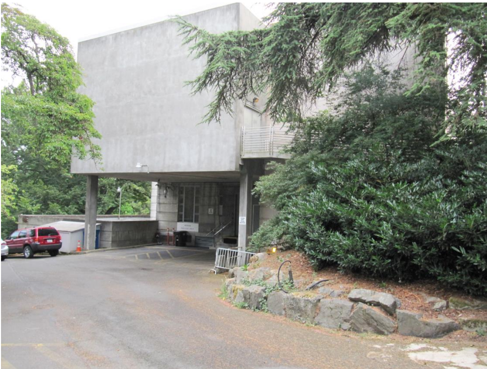
011 View looking southeast at driveway, north facade and loading dock.
