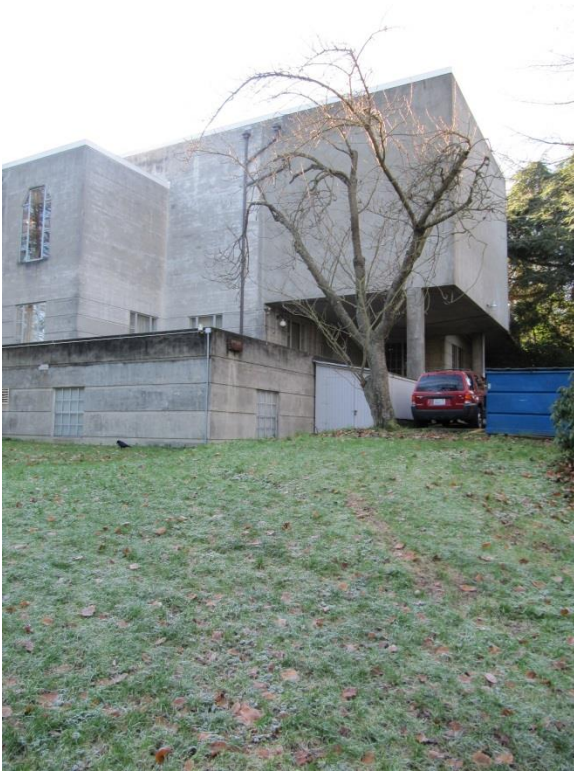
010 Oblique view looking southwest at the northeast corner and loading dock.
