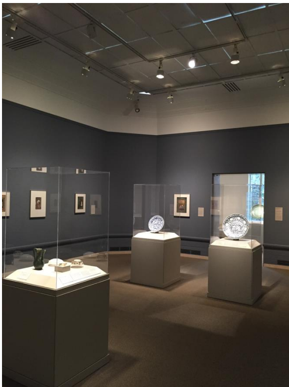
026 Typical gallery area with high vaulted ceilings. Originally ceiling grid with opaque panels now painted.
