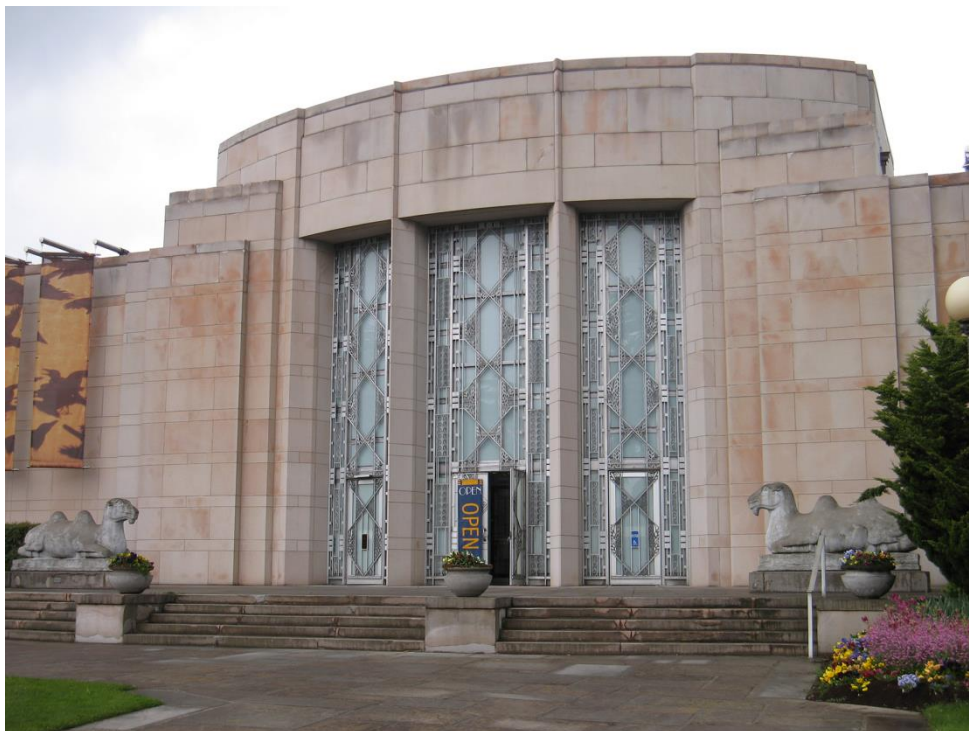
012 Detail view of the aluminum grille work at the main entry, east façade.
