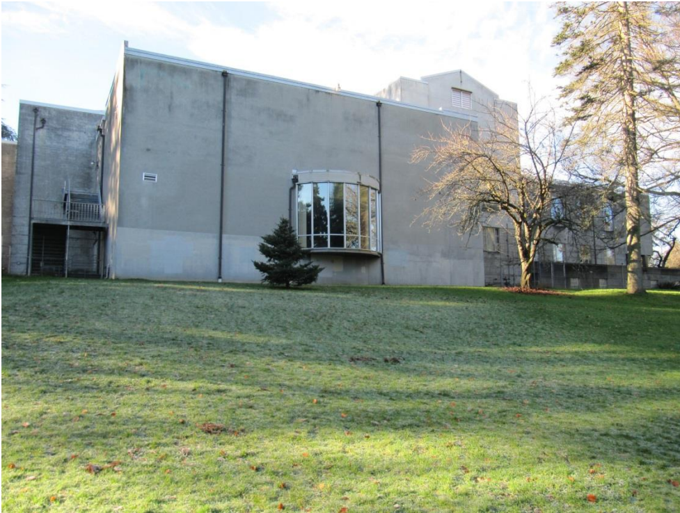
008 View looking west at the center section of the east façade.
