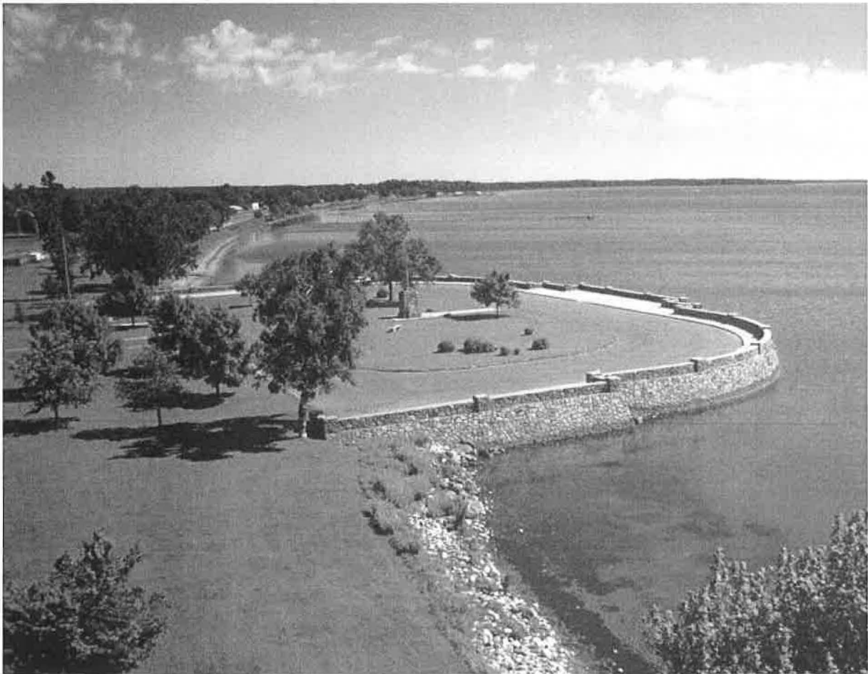
Figure 9. Since its completion in 1939, the Garrison Concourse has drawn visitors to this small community on the northwestern shore of Mille Lacs Lake. This recent photo is prominently displayed on the front page of the Garrison Commercial Club's web site (circa 2009, Garrison Commercial Club photo).
