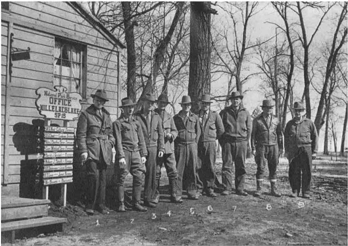
Figure 2. CCC officials and Local Experienced Men (LEMs) in front of the Mille Lacs Lake Highway Wayside CCC Camp office, part of the 15-building CCC camp located about .3-mile south of Garrison Concourse. Left to right: W. G. Neal (cultural foreman or naturalist), Don G. Chapel (landscape architect), Abe J. Sperling (chief engineer and senior foreman), Conrad Molstad (senior foreman), Harold J. Grutsch (foreman), Melburn J. Schuft (foreman), Harold E. Dickinson (junior foreman), H. T. Lane (junior foreman), and William Bowers (blacksmith). The sign board near the office door lists the men's names and positions (circa 1940, camera possibly facing northeast, Minnesota Historical Society).
