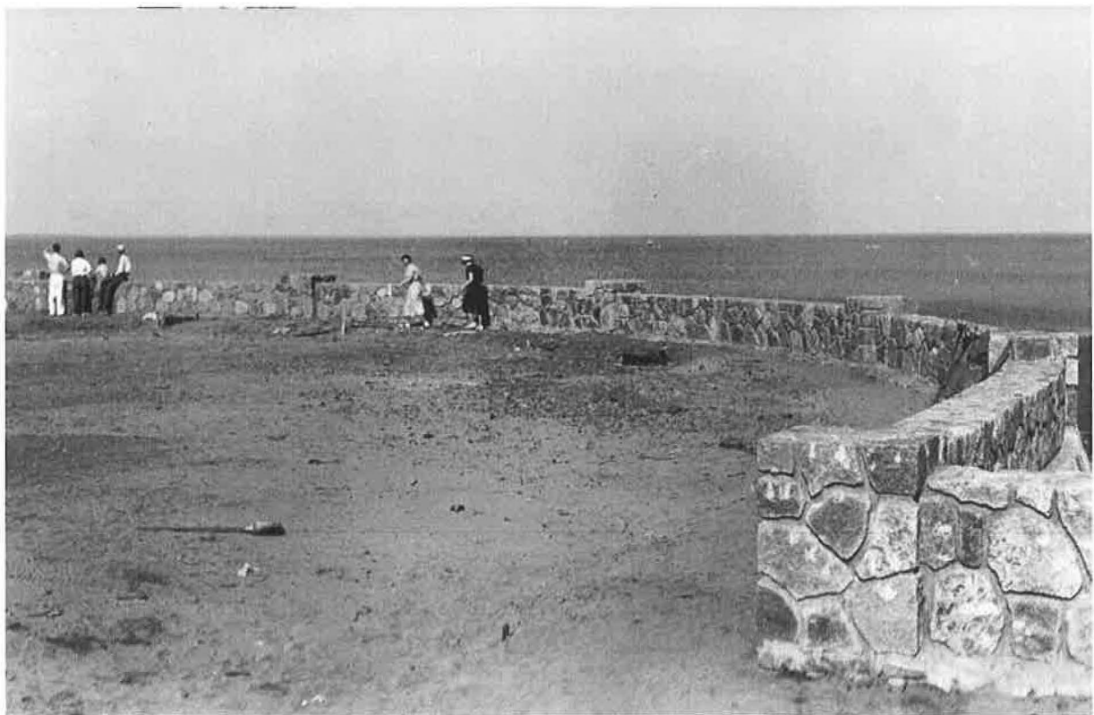
Figure 5. The concourse under construction (photo by A. R. Nichols for the Minnesota Dept. of Highways, probably summer 1937, camera facing east, Dept. of Transportation Collection, Minnesota Historical Society).
