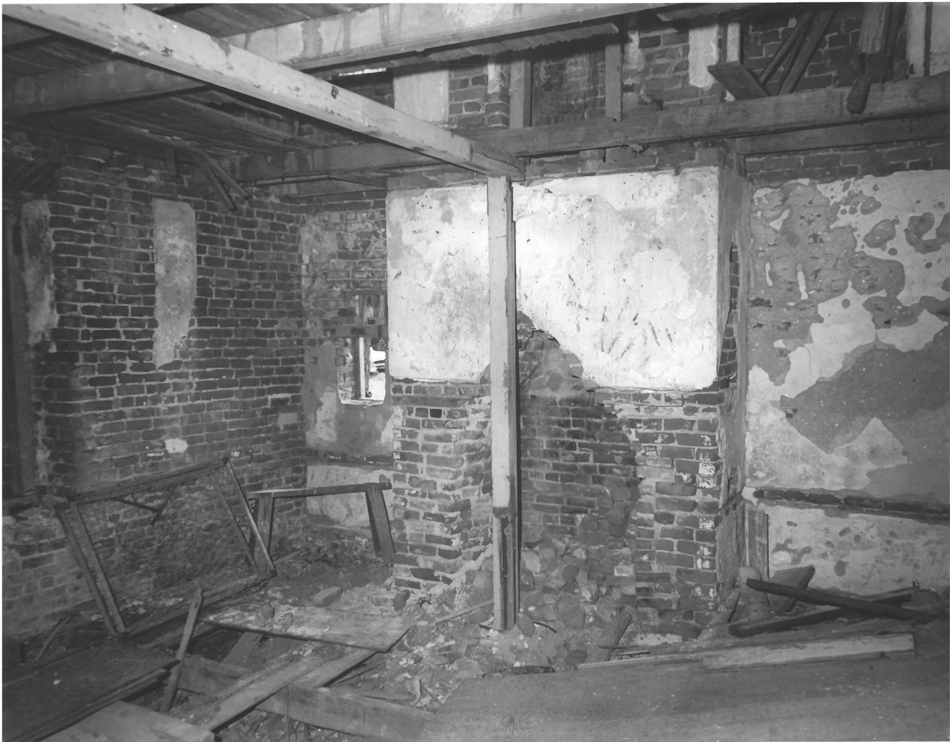
WI-9 Interior, Yellow Brick House, about 1970.
