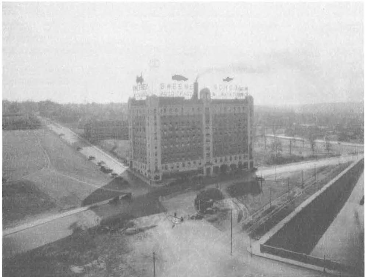
Figure 18: Exterior photograph of Sweeney Automobile and Tractor School, 1922. Source: Missouri Valley Special Collections, Kansas City Public Library, Kansas City, Missouri.
