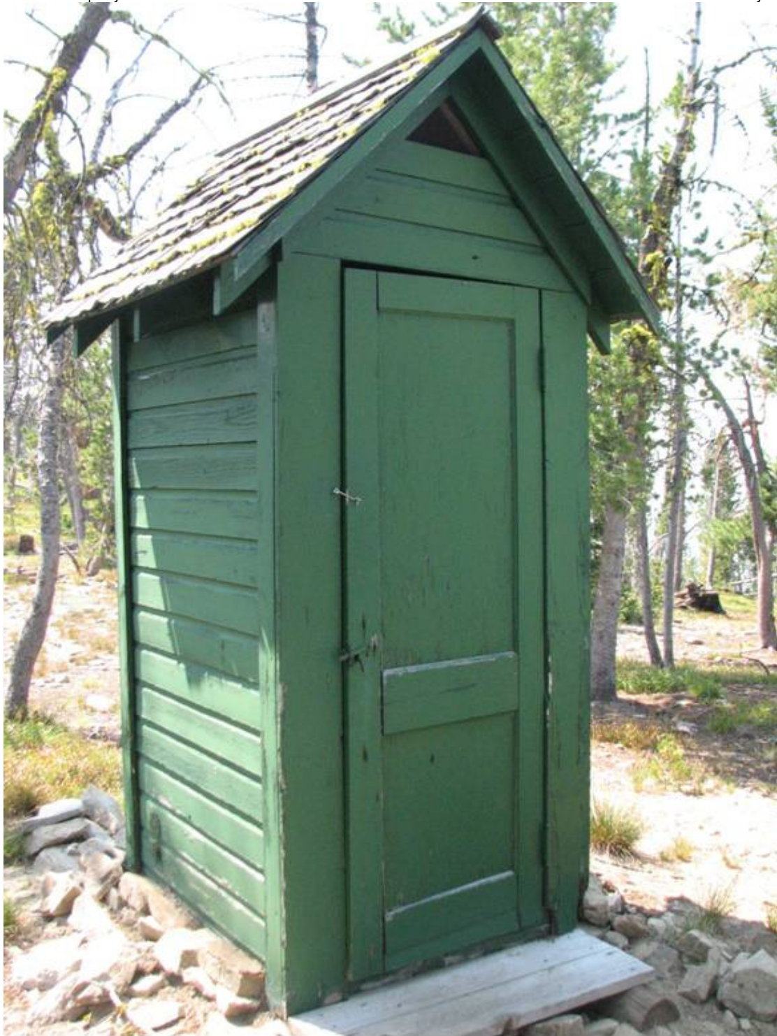
MT_RavalliCounty_MedicinePointLookout_0011. Looking southwest to the east and north walls of the outhouse.
