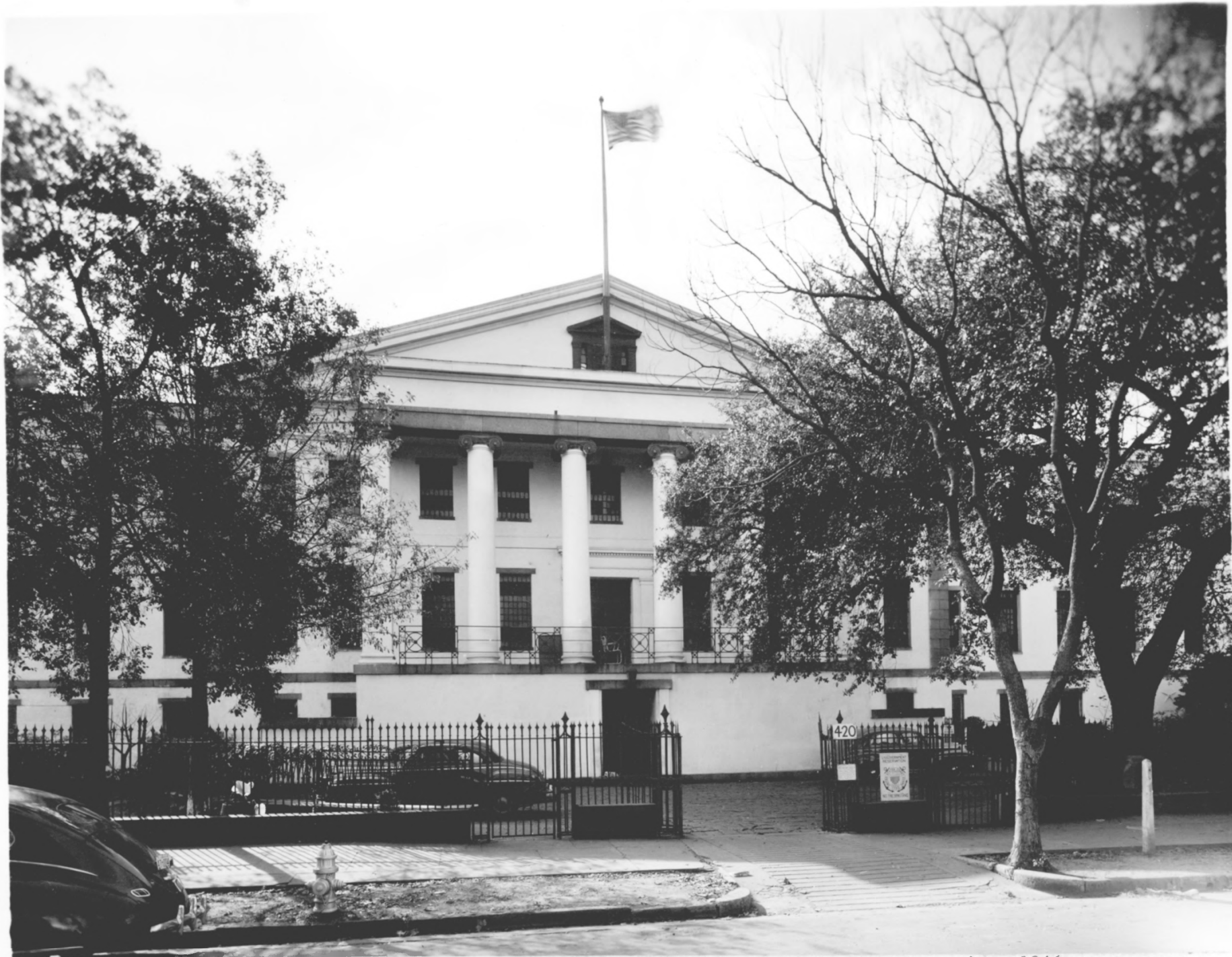
United States Branch Mint, New Orleans, Louisiana. Front facade, central portico, 1946. Photo by L. L. Martin for NPS
