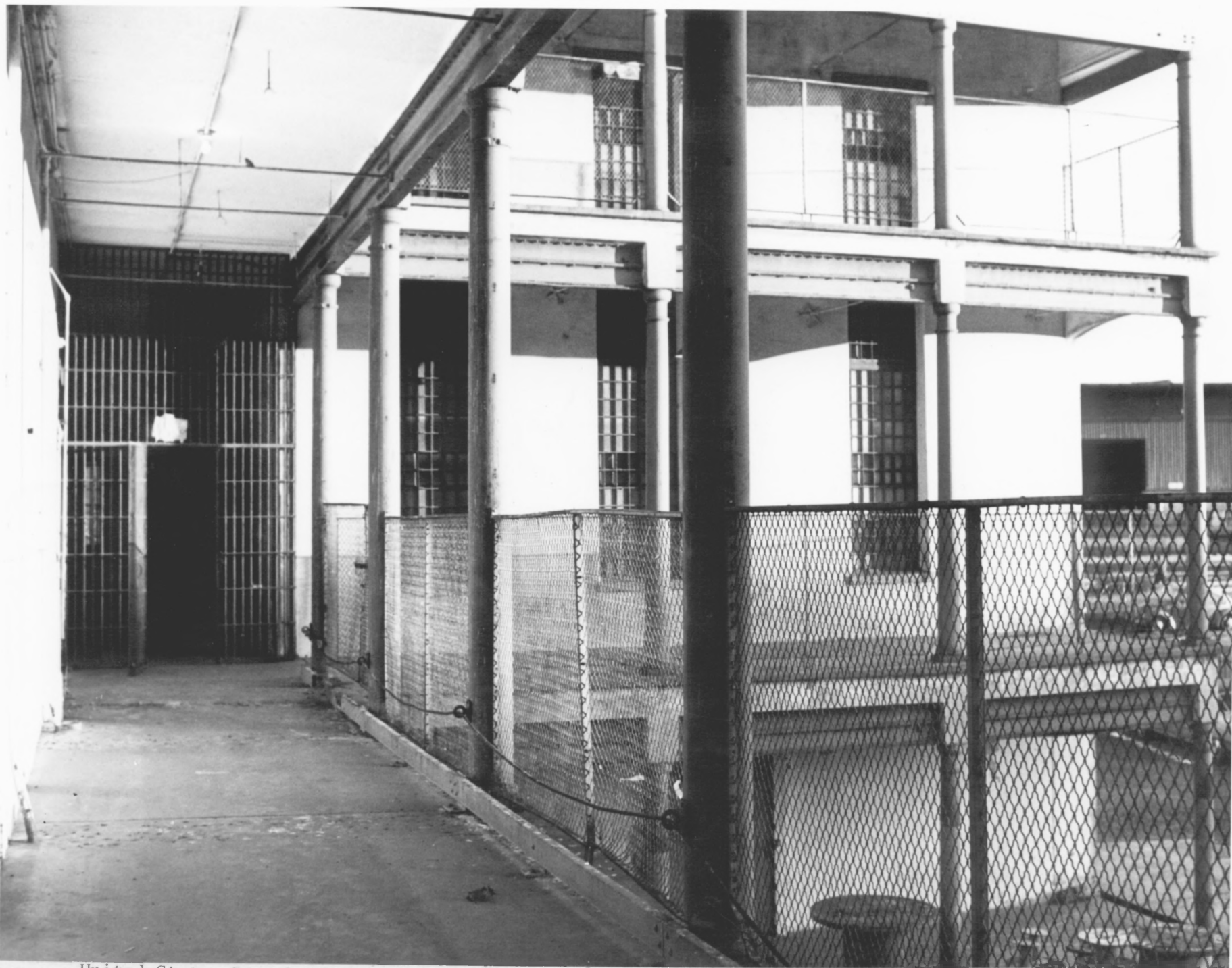
United States Branch Mint, New Orleans--Southeast Wing, showing galleries and recent jail. NPS Photo 1974
