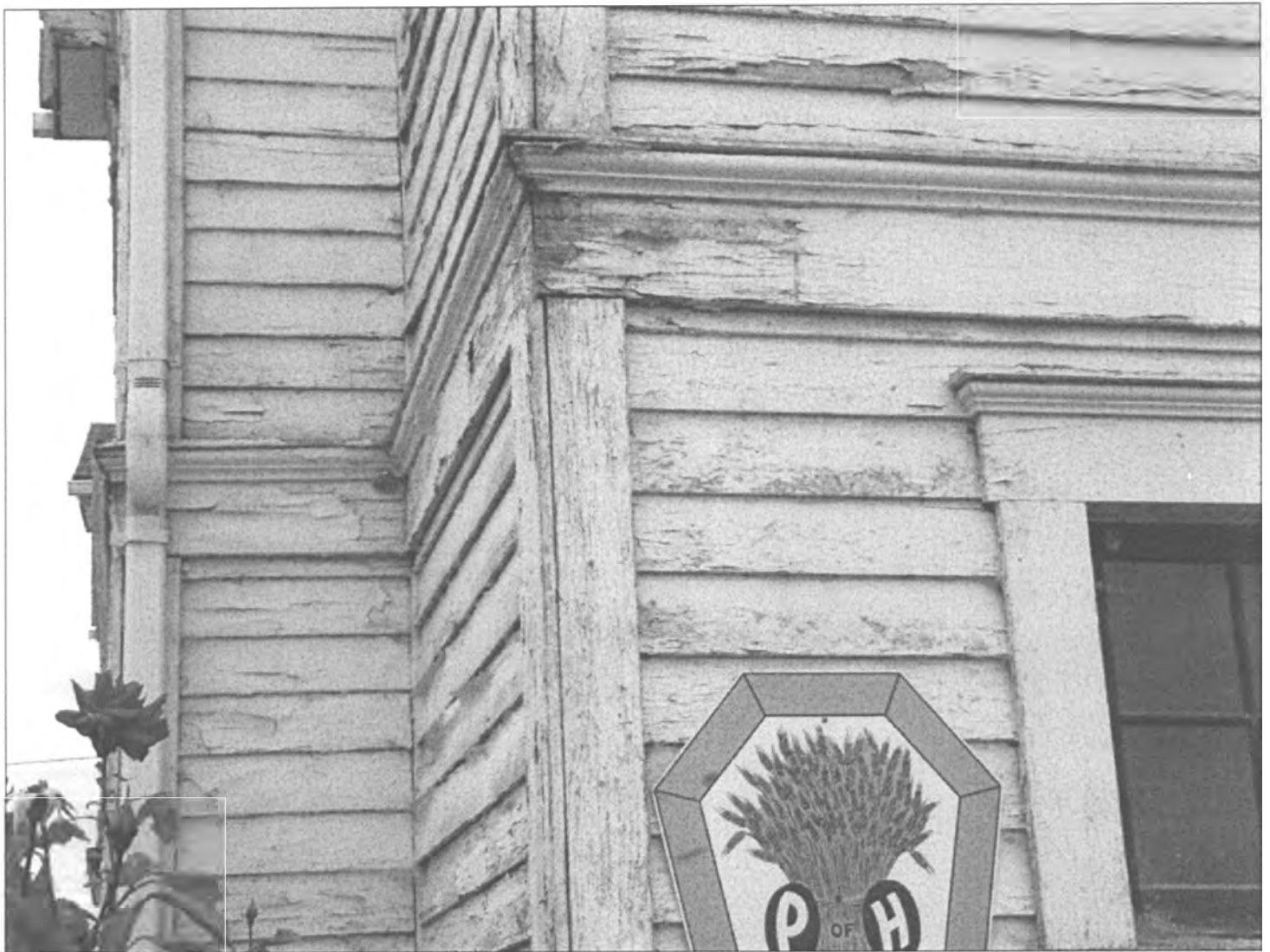
Photo 14. East elevation siding, beltcourse and window trim detail.
