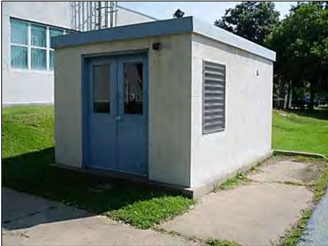
Figure 3. Mechanical Equipment Building, Army Publications Distribution Center
