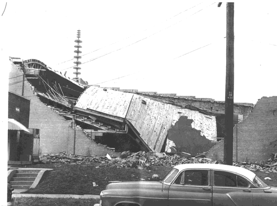
Photograph of the Kessler Theater following the April 1957 Tornado, showing collapsed roof and damage to south façade.
