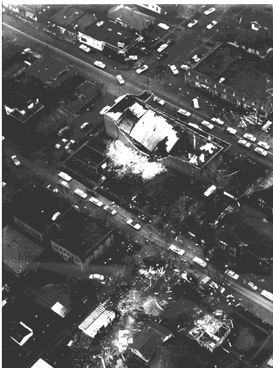
Aerial view of the tornado's path, including roof and wall damage to the Kessler Theater Camera facing northwest Dallas Morning News , April 3, 1957
