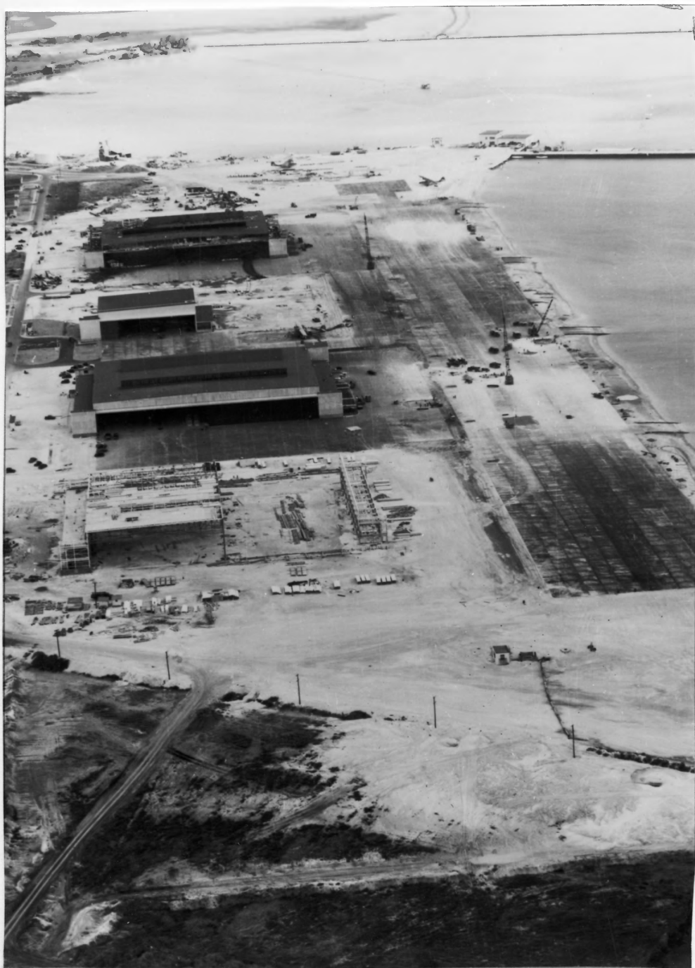
Aerial of Kaneohe Naval Air Station following the Japanese attack. Hangar No. 1, at top of photo, was burned out. The small structure immediately below it was later replaced with Hangar No. 2. Hangar No. 3 appears not to have been damaged. Hangar No. 4, at the bottom of the photo, was still under construction.
