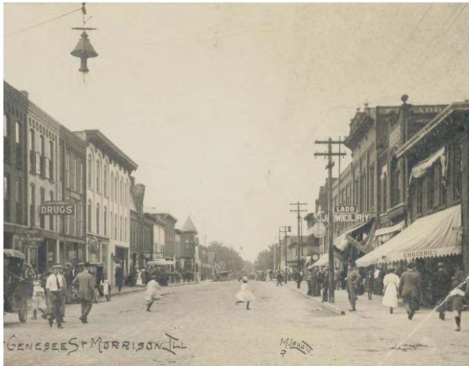
Figure 7. Morrison, Illinois, 100 block of West Main Street, looking west (1912).
