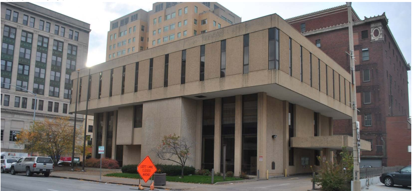
Figure 17: Citizens Federal Savings and Loan, 101 West 3 rd Street, 2014. Source: Lauren Rieke.
