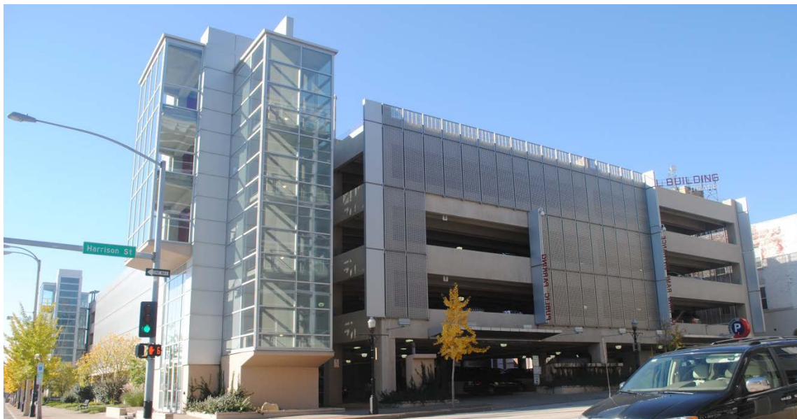
Figure 11: Harrison Street Parking Ramp, 202 Harrison Street, 2014. Source: Lauren Rieke.
