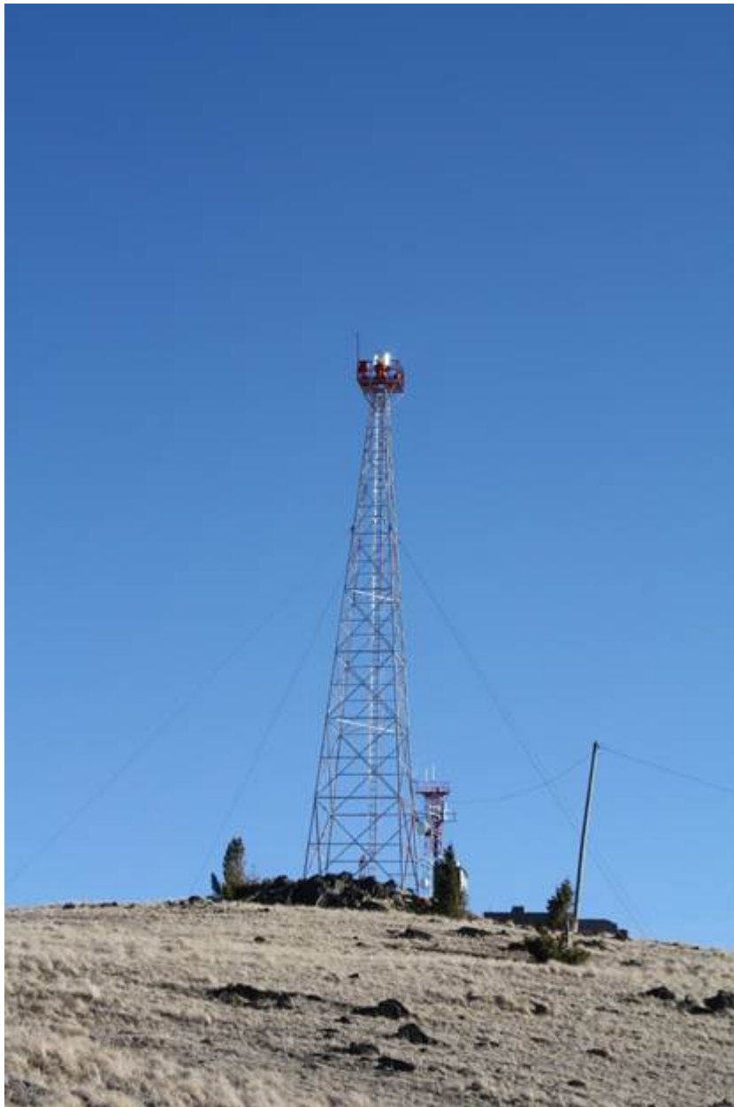
Photo #0001: MacDonald Pass Airway Beacon with beacon in foreground. View to the South. Photo date: April 1, 2013.
