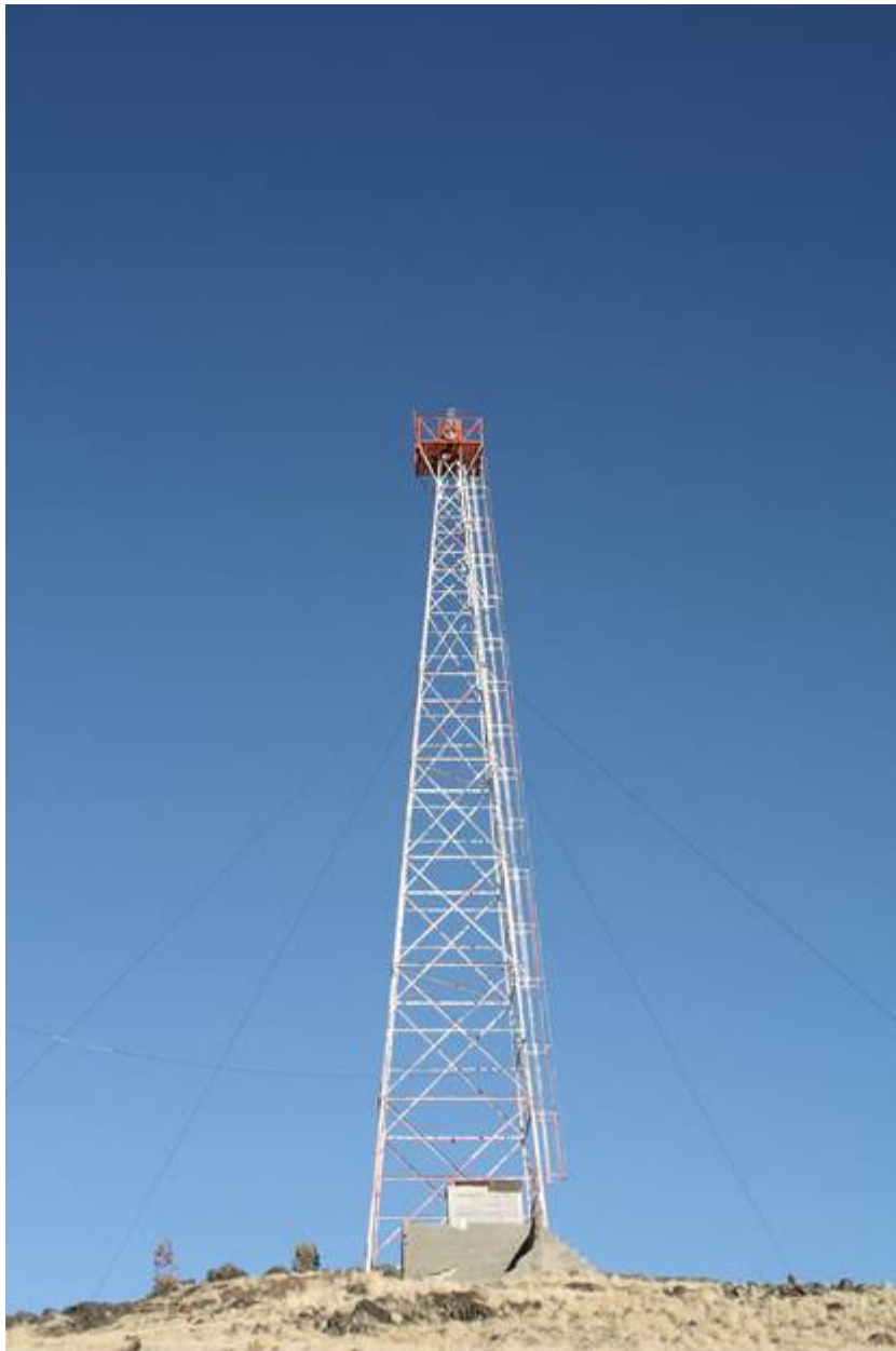
Photo #0002: MacDonald Pass Airway Beacon with generator house foundation in foreground. View to the east. Photo date: April 1, 2013.
