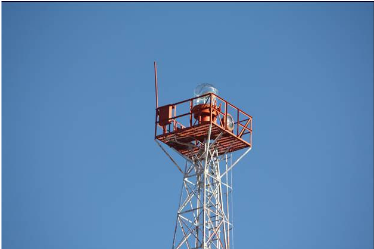
Photo #0005: MacDonald Pass Airway Beacon. Close up of dome and platform at top of beacon, view to southeast. Photo date: April 1, 2013.
