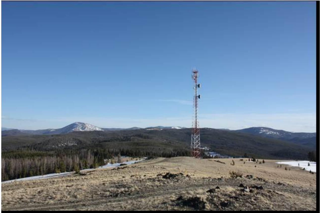
Photo #0010: MacDonald Pass Airway Beacon. Overview of property. View to the south. Photo date: April 1, 2013.
