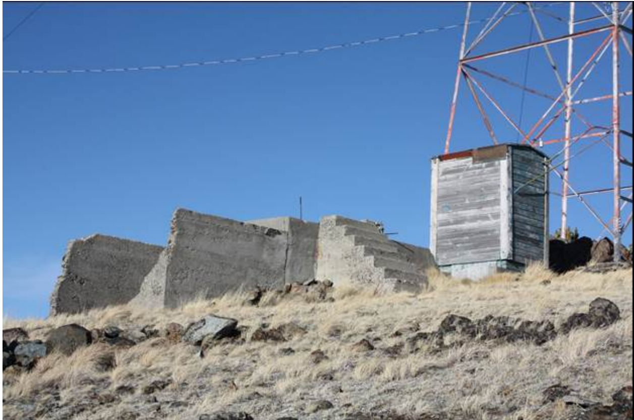
Photo #0007: MacDonald Pass Airway Beacon. Left to right: generator house foundation, electrical shed, southwest corner of beacon tower. View to the northeast. Photo date: April 1, 2013.
