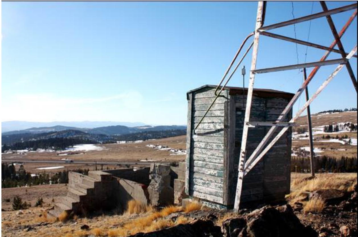
Photo #0006: MacDonald Pass Airway Beacon. Left to right: generator house foundation, electrical shed, southwest corner of beacon tower. View to the northwest. Photo date: April 1, 2013.
