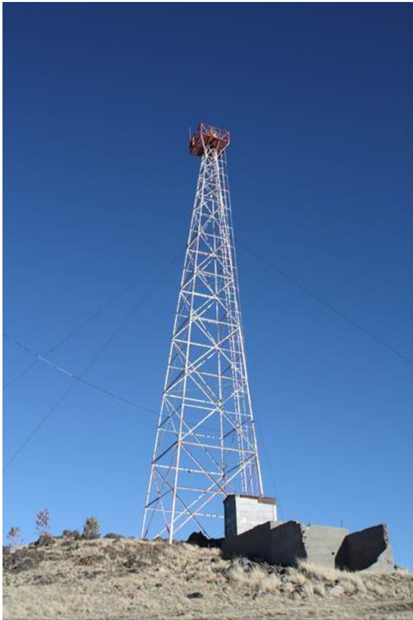
Photo #0008: MacDonald Pass Airway Beacon. Generator house foundation in foreground, electrical shed behind generator house foundation, beacon behind electrical shed. View to the east-southeast. Photo date: April 1, 2013.
