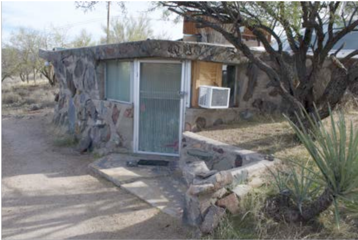
AZ_Maricopa County_Dome House_0004
