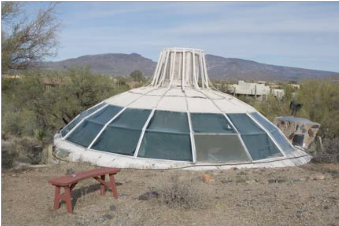
AZ_Maricopa County_Dome House_0002
