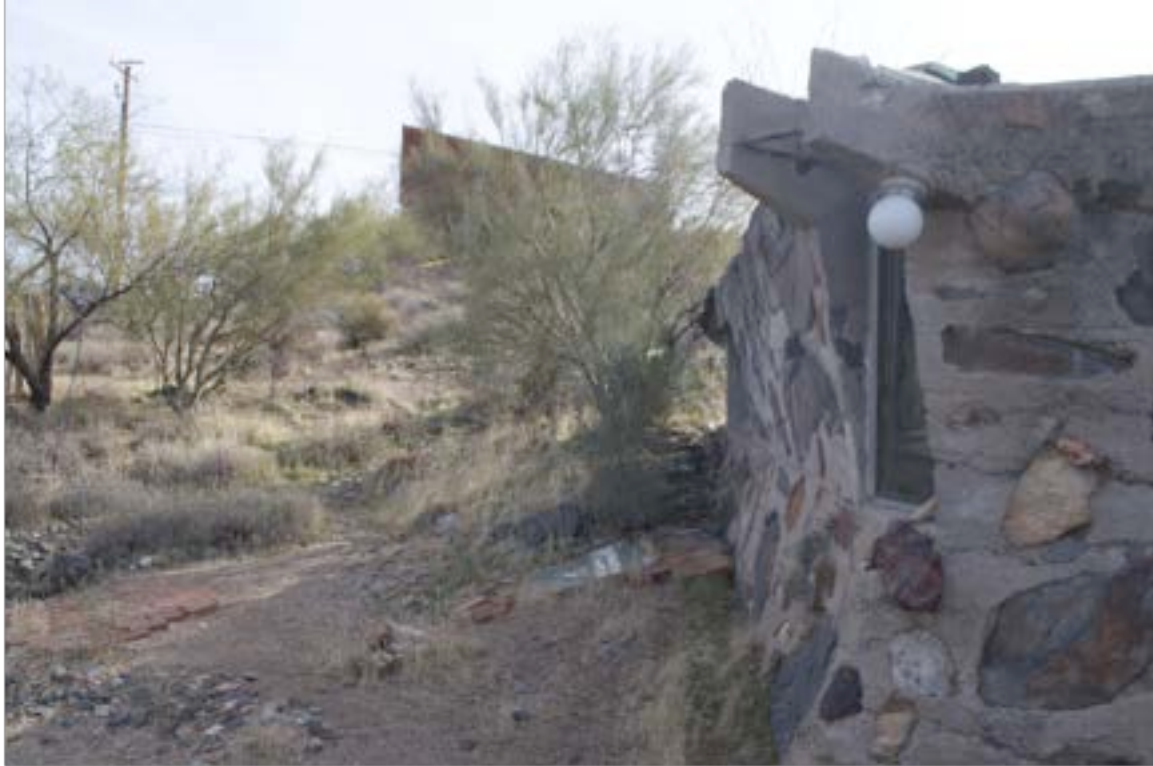
AZ_Maricopa County_Dome House_0006
