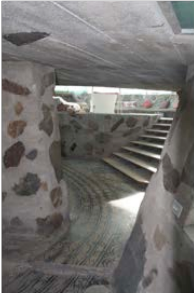
AZ_Maricopa County_Dome House_0007
