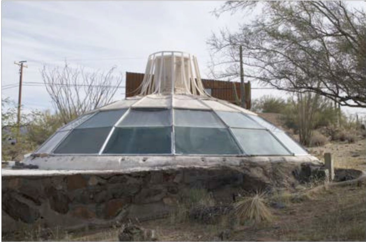
AZ_Maricopa County_Dome House_0001
