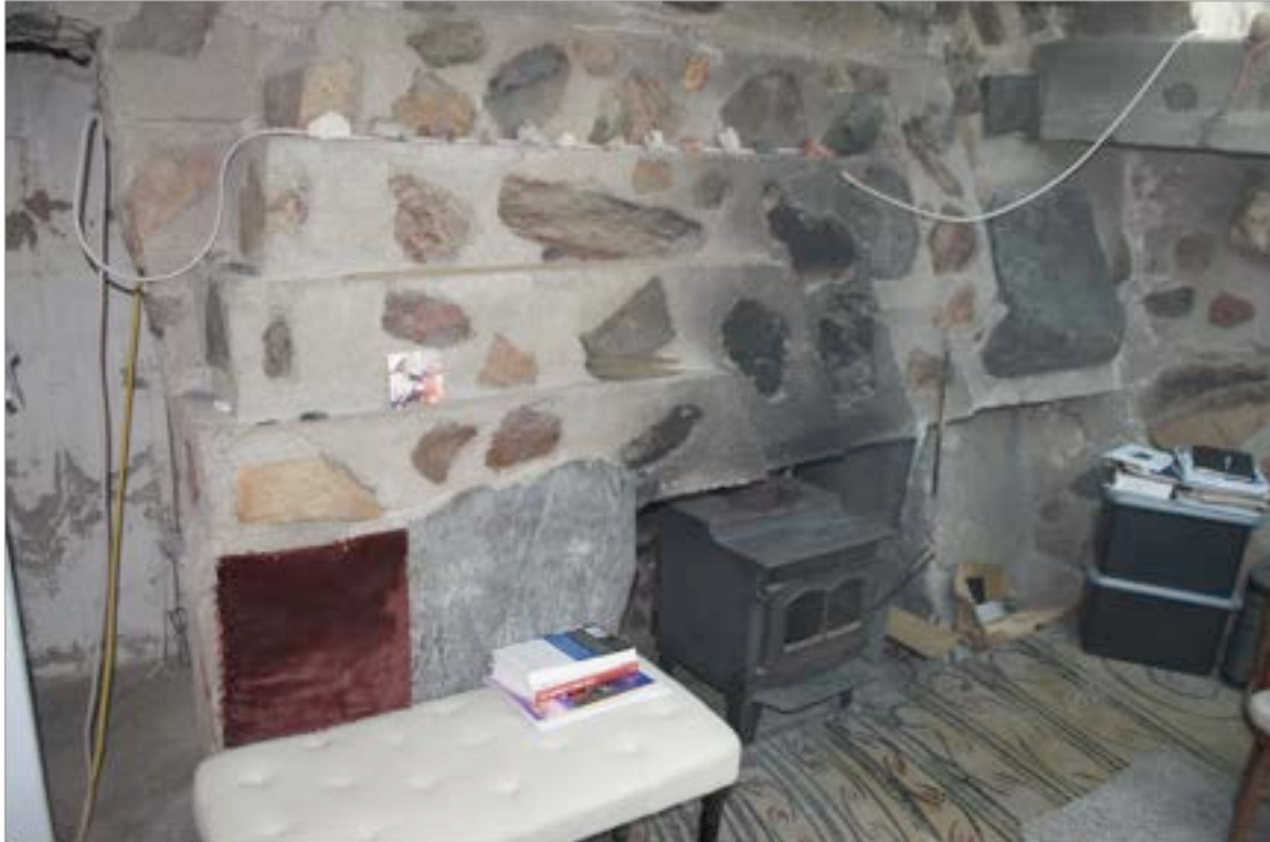
AZ_Maricopa County_Dome House_0012
