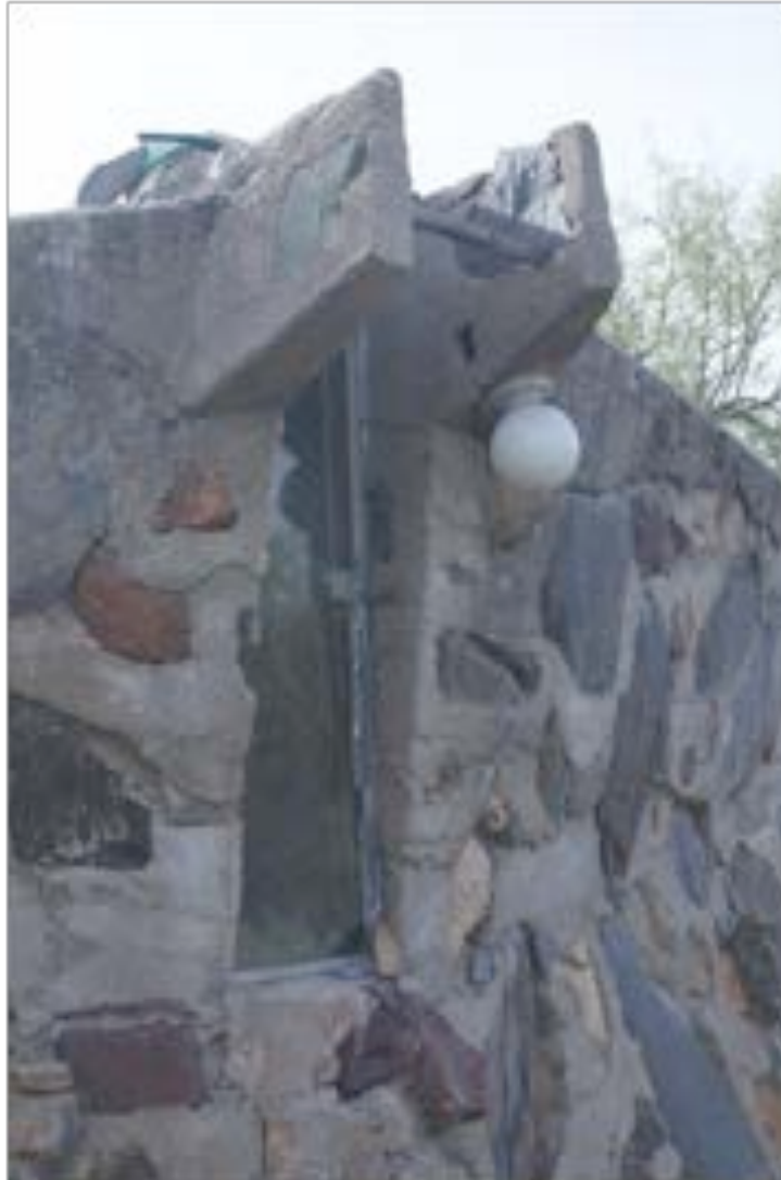
AZ_Maricopa County_Dome House_0005
