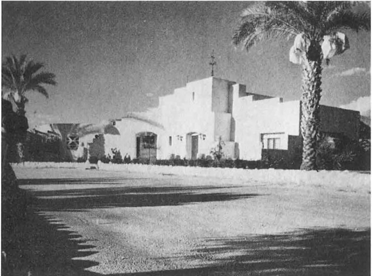
Figure 4. Ferguson House, Front Elevation, Anonymous Photograph, c 1938.
