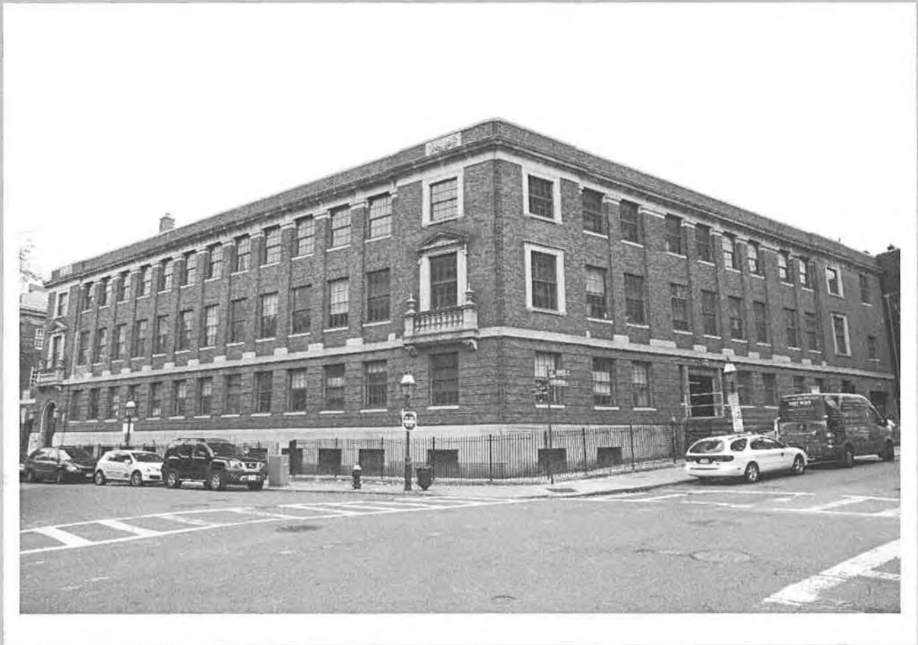
6. East and north elevations, Boston Printing Department Building, camera facing southwest.
