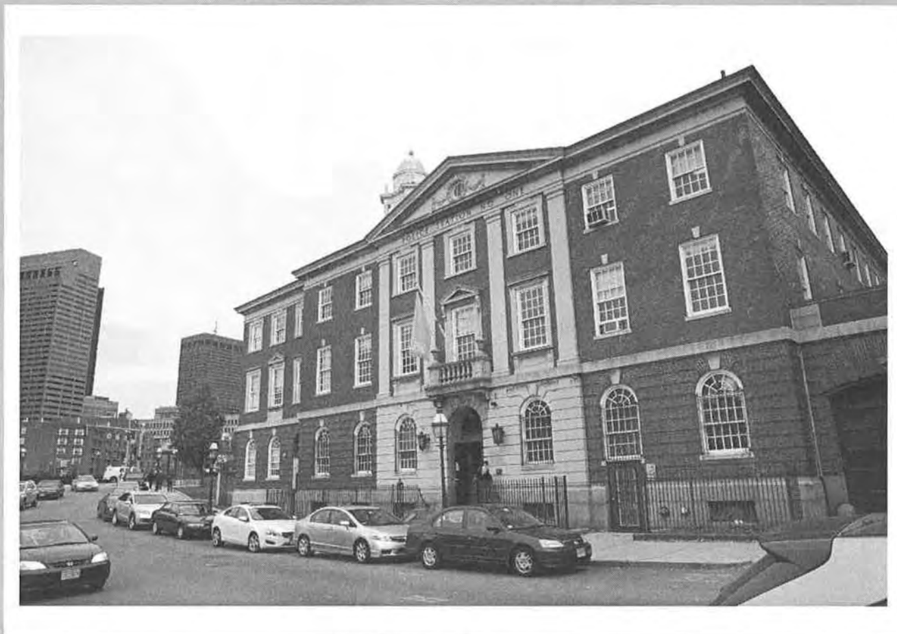
4. East and north elevations, Police Station Number One, camera facing southwest.
