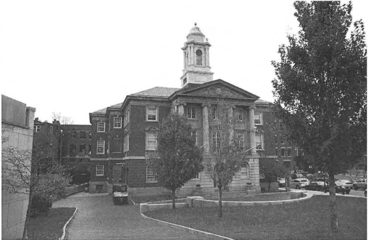
2. West and south elevations, camera facing northeast.
