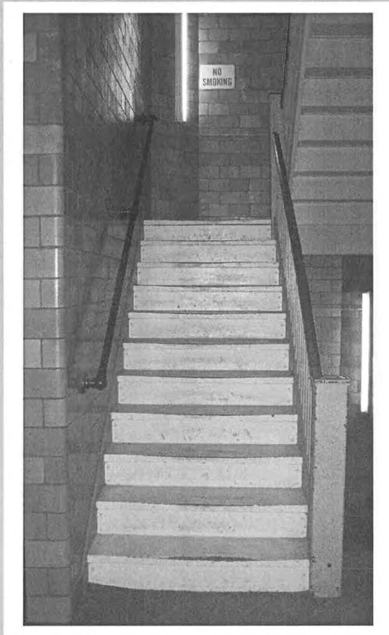
11. Printing Department Building, stair detail.
