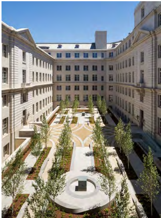
Photo 10. View of courtyard, looking east (Blake Marvin—HKS, Inc., May 2013)
