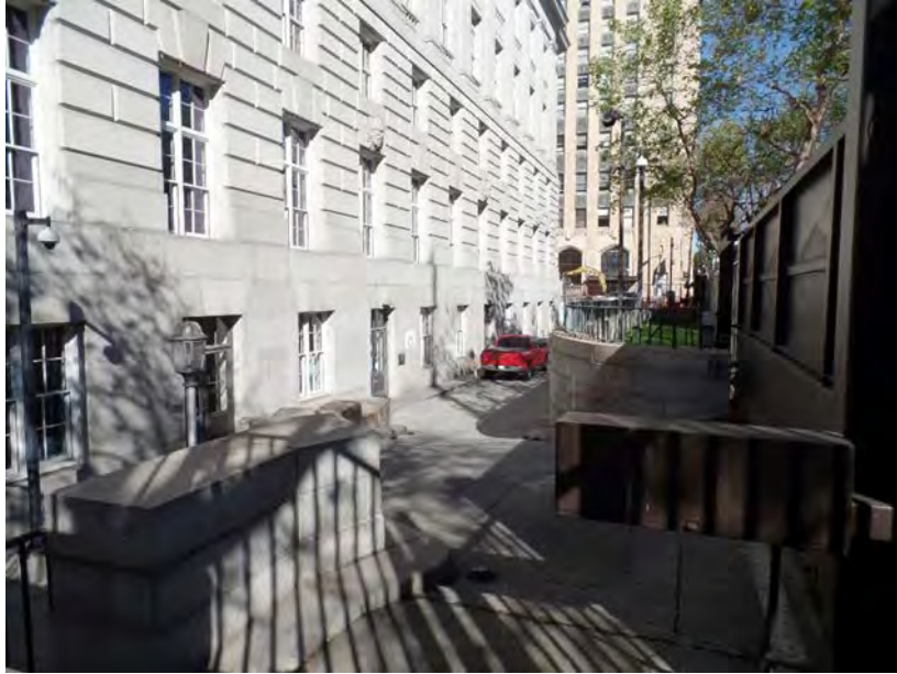
Photo 9. Partial view of east elevation with sunken basement access area (Garavaglia Architecture, Inc., February 2015)
