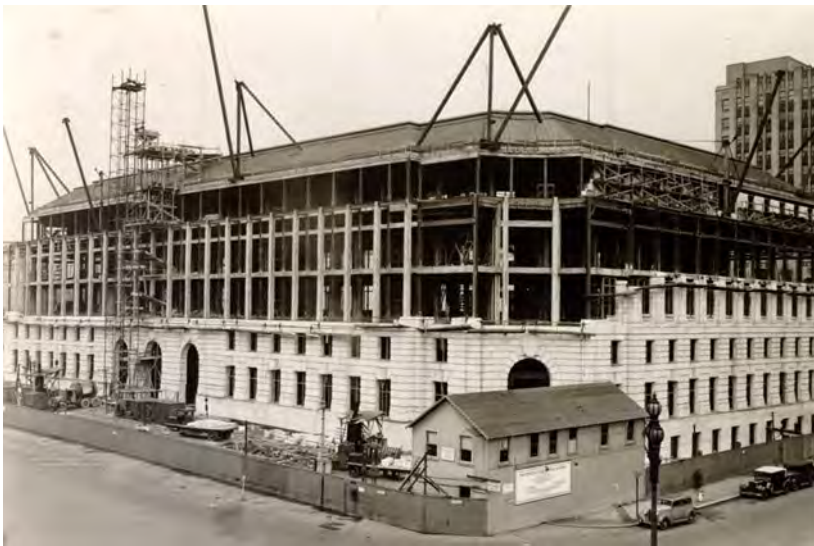
Figure D. Granite cladding takes place, January 1935 (San Francisco History Center, San Francisco Public Library)
