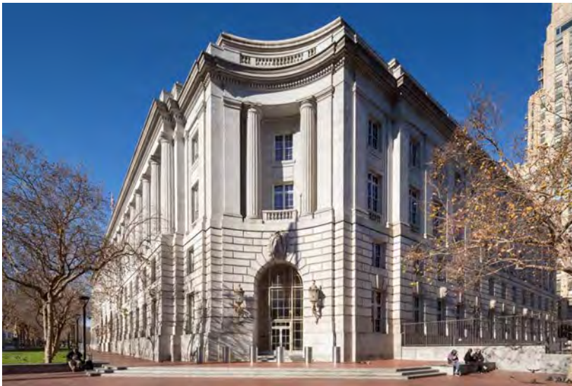
Photo 2. Southeast corner, showing overall facade massing elements (Blake Marvin—HKS, Inc., December 2013)
