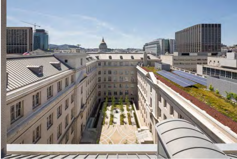
Photo 3. View of sloped sections of Main Roof at center and left and North Roof at right, looking west (Blake Marvin—HKS, Inc., May 2013)
