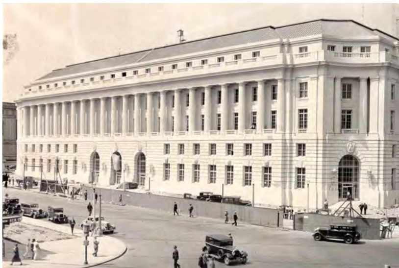
Figure F. Construction of 50 UNP nearing completion, view from Fulton Street, April 1936 (San Francisco History Center, San Francisco Public Library)
