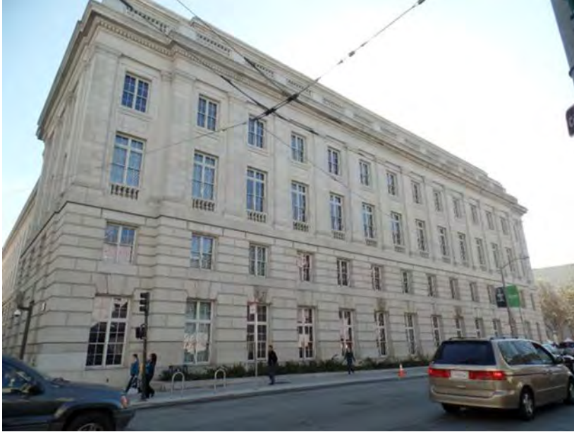
Photo 7. View of west elevation (Garavaglia Architecture, Inc., February 2015)
