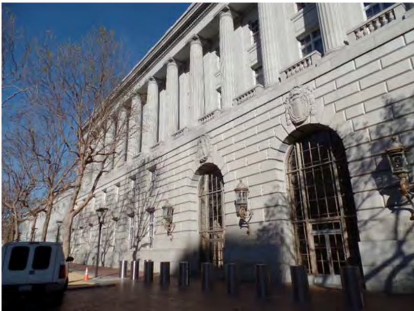
Photo 4. Partial view of south façade (Garavaglia Architecture, Inc., February 2015)
