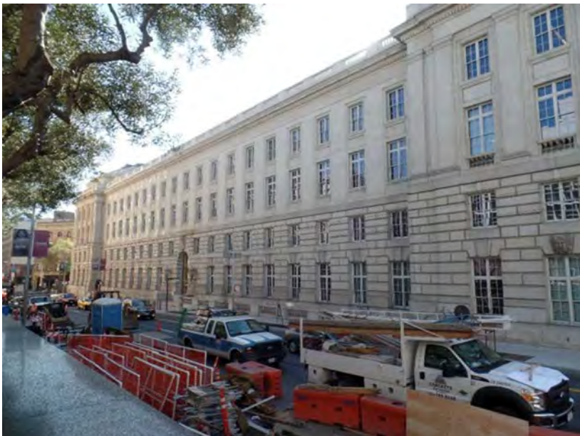
Photo 8. Partial view of north elevation (Garavaglia Architecture, Inc., February 2015)
