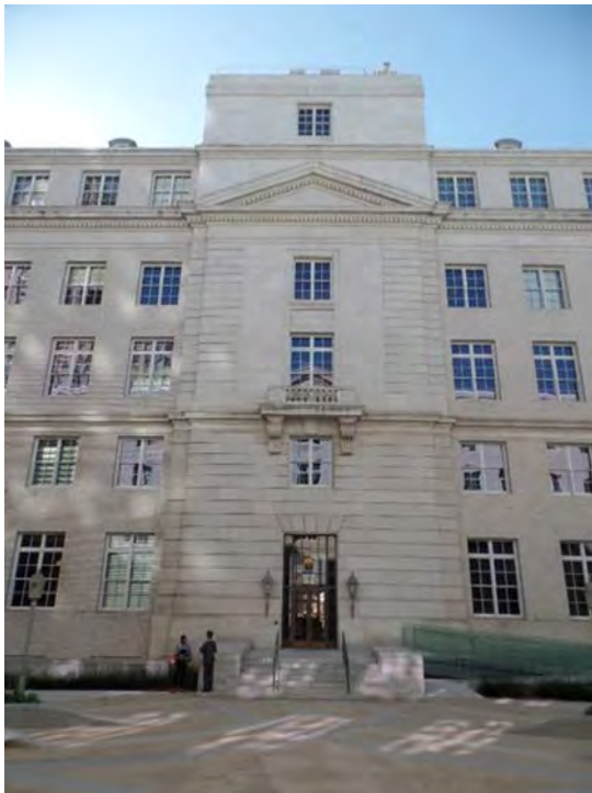
Photo 12. View of courtyard entrance to south elevator lobby (Garavaglia Architecture, Inc., February 2015)
