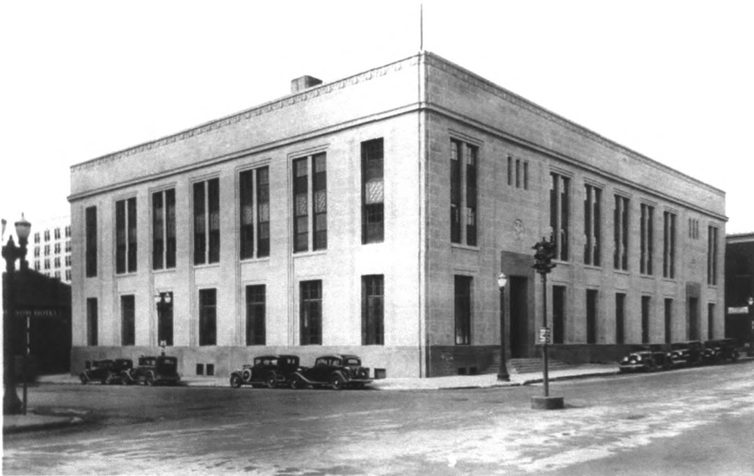
Figure 1 The United States Post Office and Court House nearly completed, circa 1933. The photographer is looking southwest and standing at the northeast corner of Perry Street (on the left) and East 4th St. (foreground and to the right). Especially noticeable in this view is the building's dark gray band of granite at ground level and around the two north entrances. The non-extant Windsor Hotel is visible at the left edge of this view. (General Services Administration)
