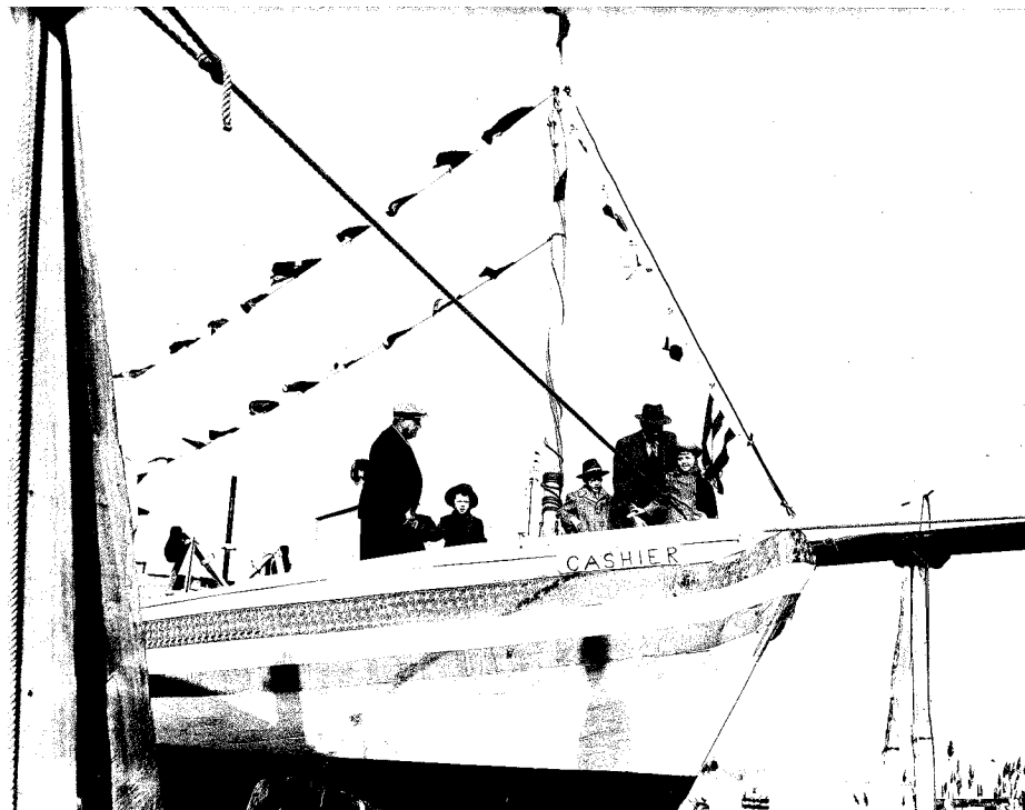
Historic Photograph #6: Relaunching of CASHIER, 1949.
