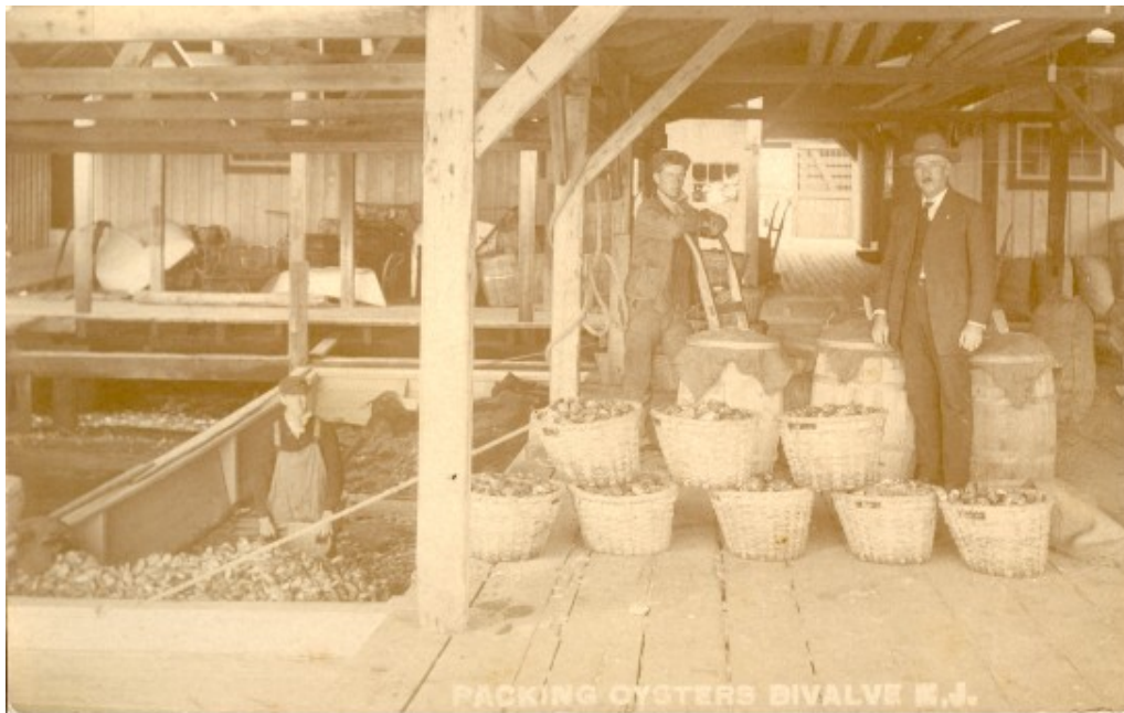
Photo #2: Oyster Shipping Sheds, wharves, early 1900's.
