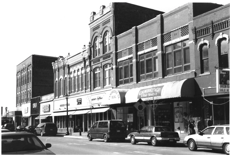
Streetscape, 3rd St. Between Center & La Fayette Winona Commercial Historic District Winona, Co., Mn Q13338-4
