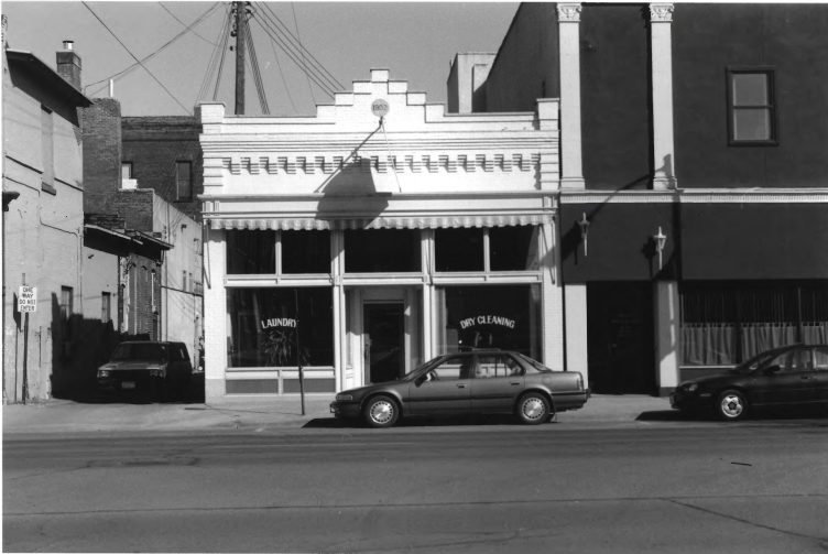
Commercial Building 164 Main St. Winona Commercial Historic District Winona Co., MN 013338-11
