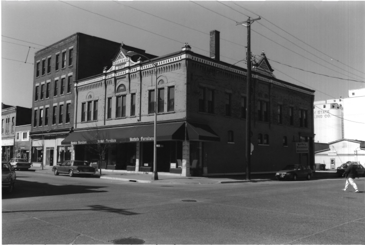
Left: Stott & Sons Bldg., 220 E. 3rd St., Right: Stott Bldg., 222-226 E. 3rd. St. Winona Commercial Historic District Winona Co., MN
