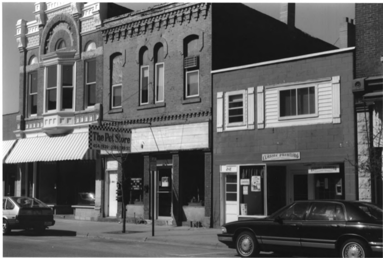
Vetkins Bldg., Commercial Bldg., & Commercial Bldg., 214, 216 & 218 E. 3rd. St. Winona Commercial Historic District Winona Co., Mn 013340-24
