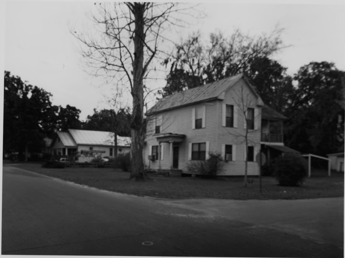
WEST DARIEN HISTORIC DISTRICT MCINTOSH COUNTY, GEORGIA PHOTOGRAPH 18 of 37
