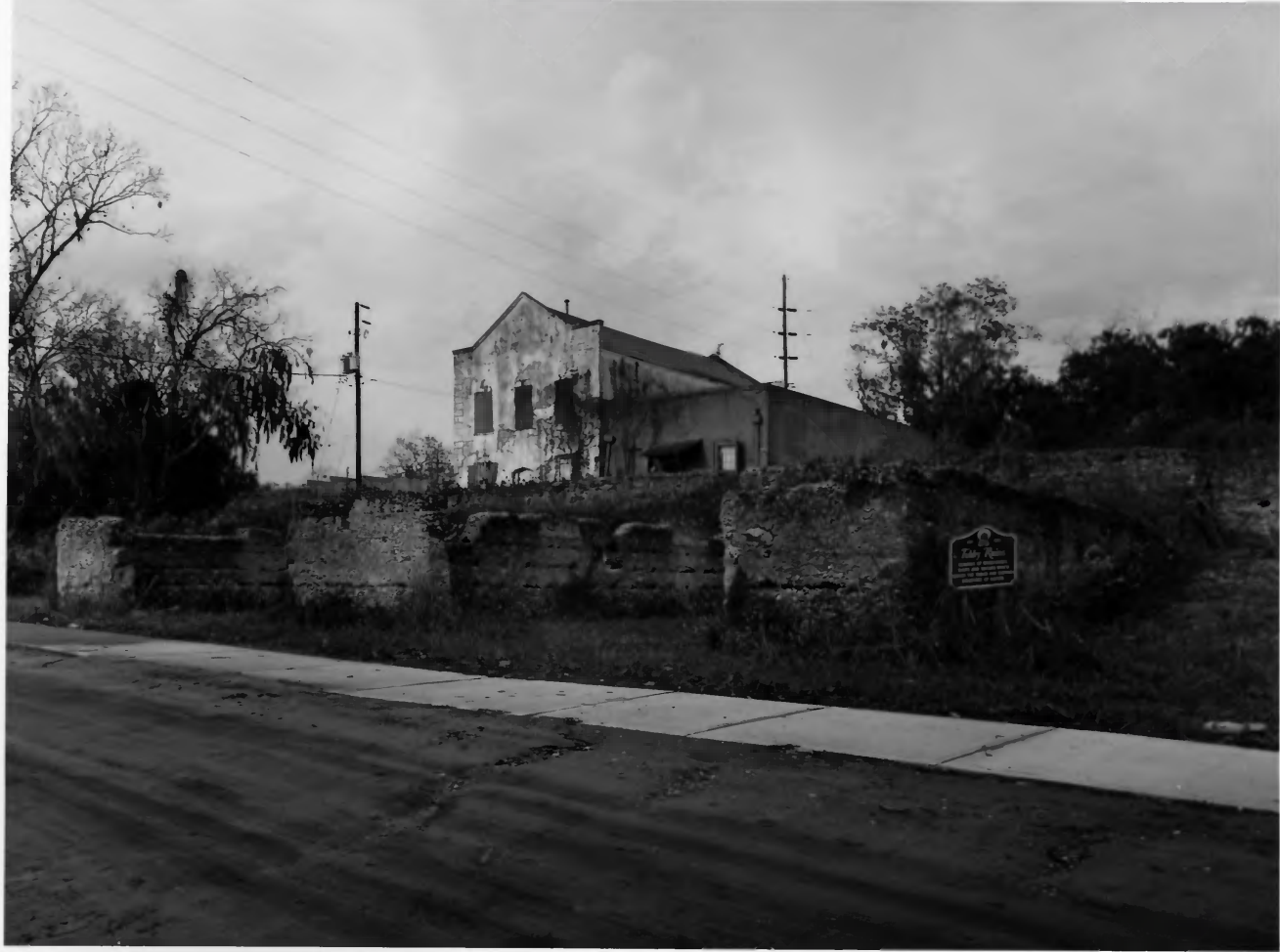
WEST DARIEN HISTORIC DISTRICT MCINTOSH COUNTY, GEORGIA PHOTOGRAPH 2 OF 37
