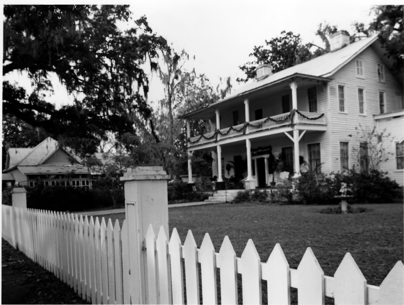
WEST DARIEN HISTORIC DISTRICT MCINTOSH COUNTY, GEORGIA PHOTOGRAPH 8 OF 37
