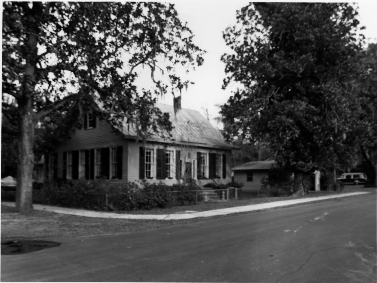
WEST DARIEN HISTORIC DISTRICT MCINTOSH COUNTY, GEORGIA PHOTOGRAPH 11 OF 37
