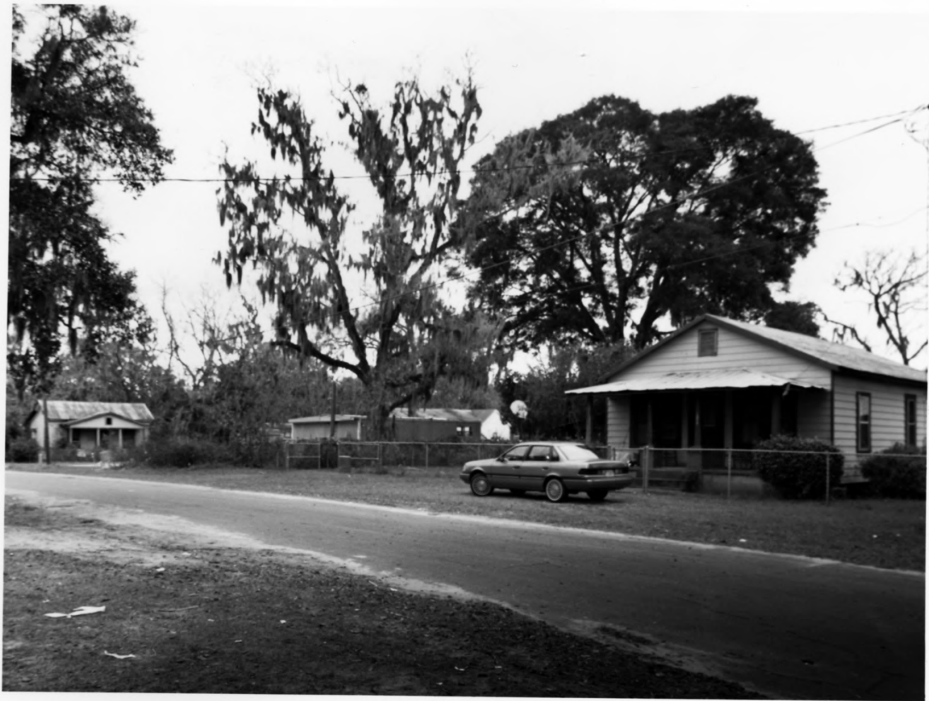
WEST DARIEN HISTORIC DISTRICT MCINTOSH COUNTY, GEORGIA PHOTOGRAPH 35 OF 37
