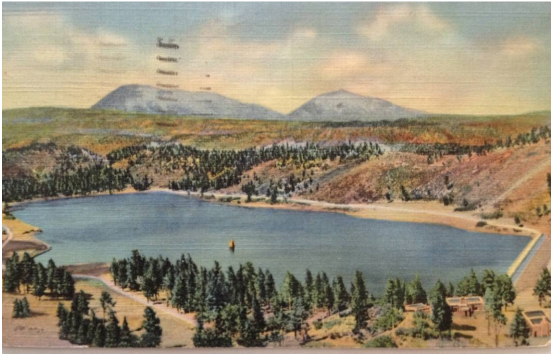
Figure 9: View of Monument Lake Park showing Kendall House (Building 1) and El Miramonte Lodge (Building 2) in lower right; Spanish Peaks in distance, circa 1940s
