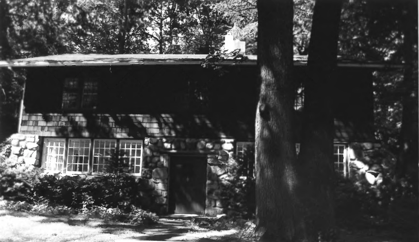
Craftsman Farms, Parsippany, N.J. 16 Manor Lane (Bakery, No.10) Photo: R.B. Benton 1984
