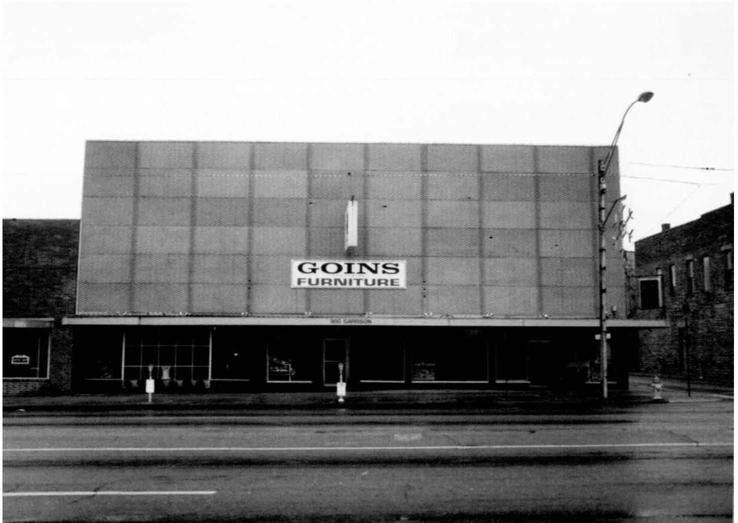
Figure 3: Arcade Department Store Building at 900 West Garrison Avenue, January 11, 1998.
