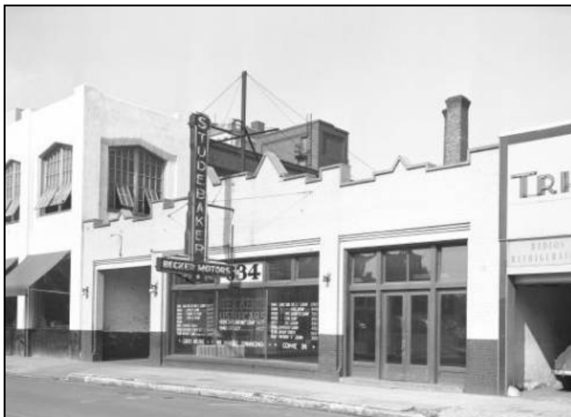
634 South 3rd Street, built by Mahan-Bowman Motor Company in 1920. Other garages stand to the left and the right. The original form is still apparent in this photograph, with a pedestrian entrance on the right, large storefront windows in the center, and a vehicle entrance on the left.
